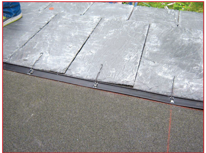
Figure 6 – Qwik Slate installation in progress. Photo courtesy of Brian Chalsma, The Roofing Company, Hampton, VA.
