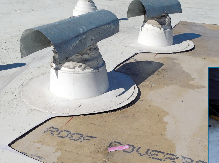
Figures 4A (left) and 4B (below) – A “wet” coverboard is shown next to 7-in. air ducts that terminate below 5-in. T-top flashings.
