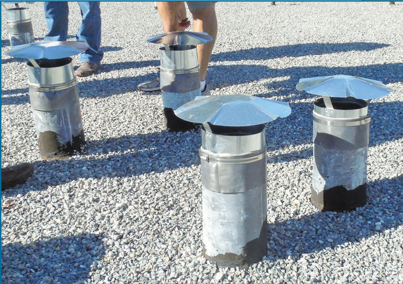
Figures 9A (right) and 9B (below) – Example of how existing low air ducts can be extended and flashed.
