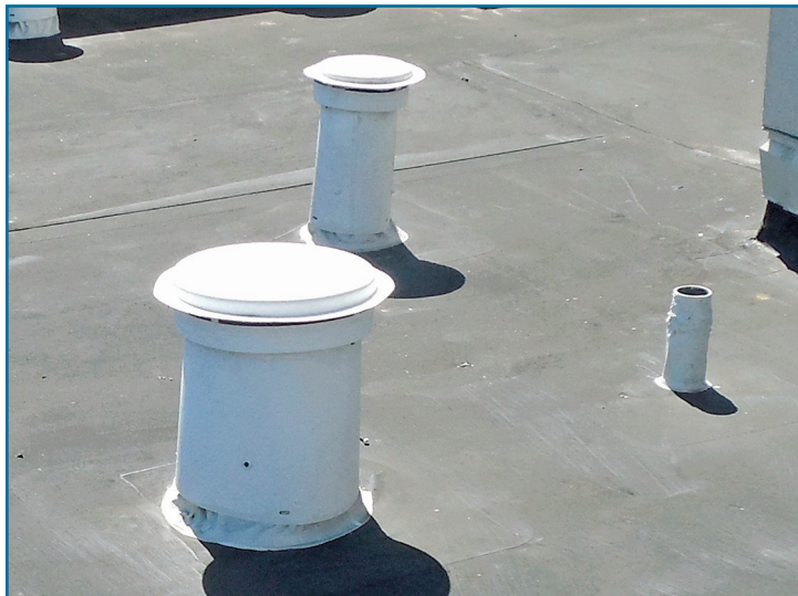
Figures 5A (above) and 5B (right) – Two air ducts are positioned in an oversized deck opening and terminated inside one large roof flashing.
