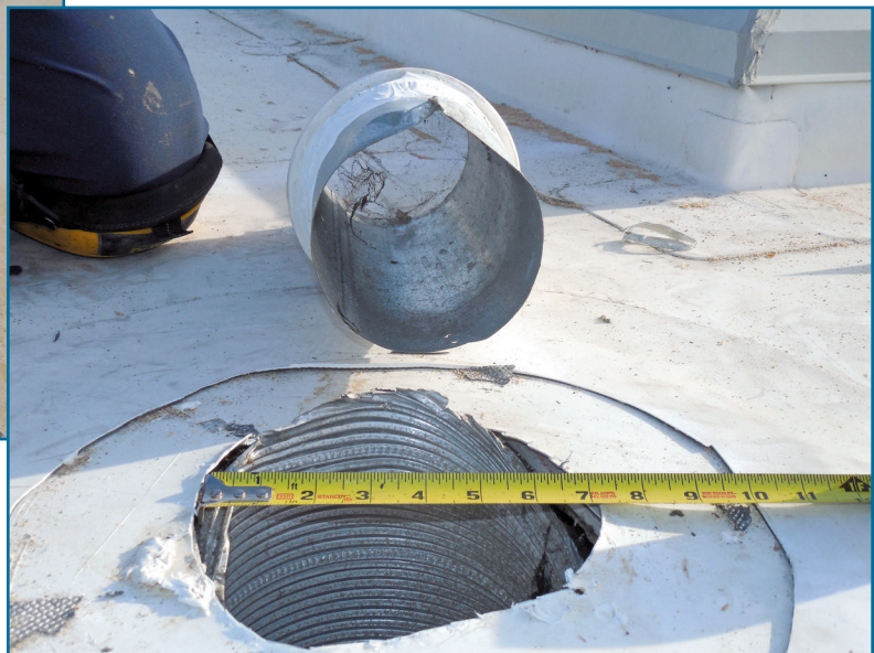
Figures 4A (left) and 4B (below) – A “wet” coverboard is shown next to 7-in. air ducts that terminate below 5-in. T-top flashings.
