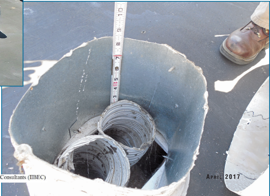
Figures 5A (above) and 5B (right) – Two air ducts are positioned in an oversized deck opening and terminated inside one large roof flashing.
