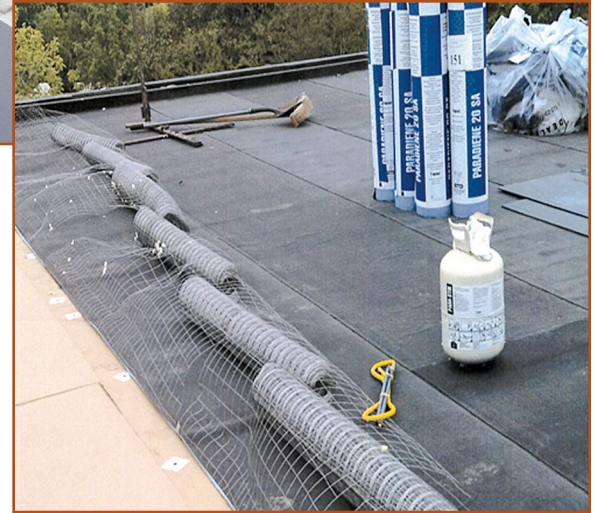
Figure 4 – In some assemblies, lightweight wire grids can be installed directly under the membrane, but due to manufacturer's concerns, they are often placed between the insulation and a coverboard.
