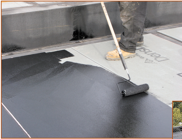
Figure 3 – Electrically conductive primer is installed directly under the membrane and meets ASTM Standard D7877.
