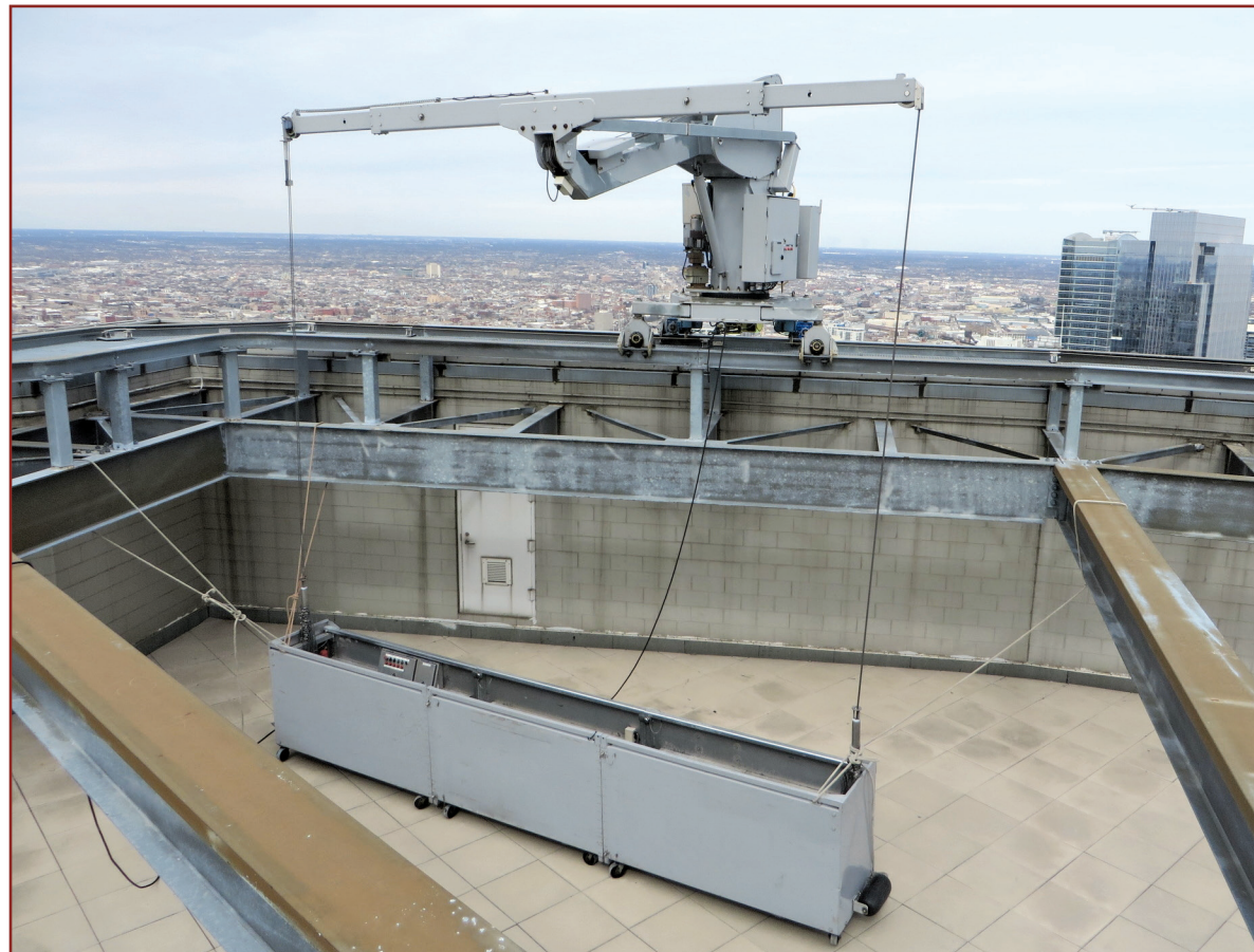
Figure 1 – Large, rail-mounted rooftop carriage.
