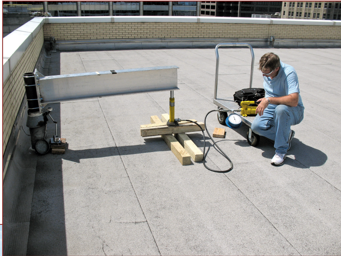
Figure 4 – Load testing of a davit base.
