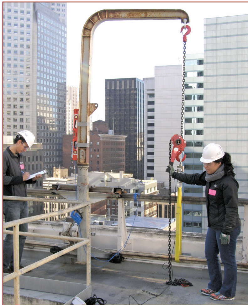
Figure 6 – Load testing of a davit mounted on a carriage.
