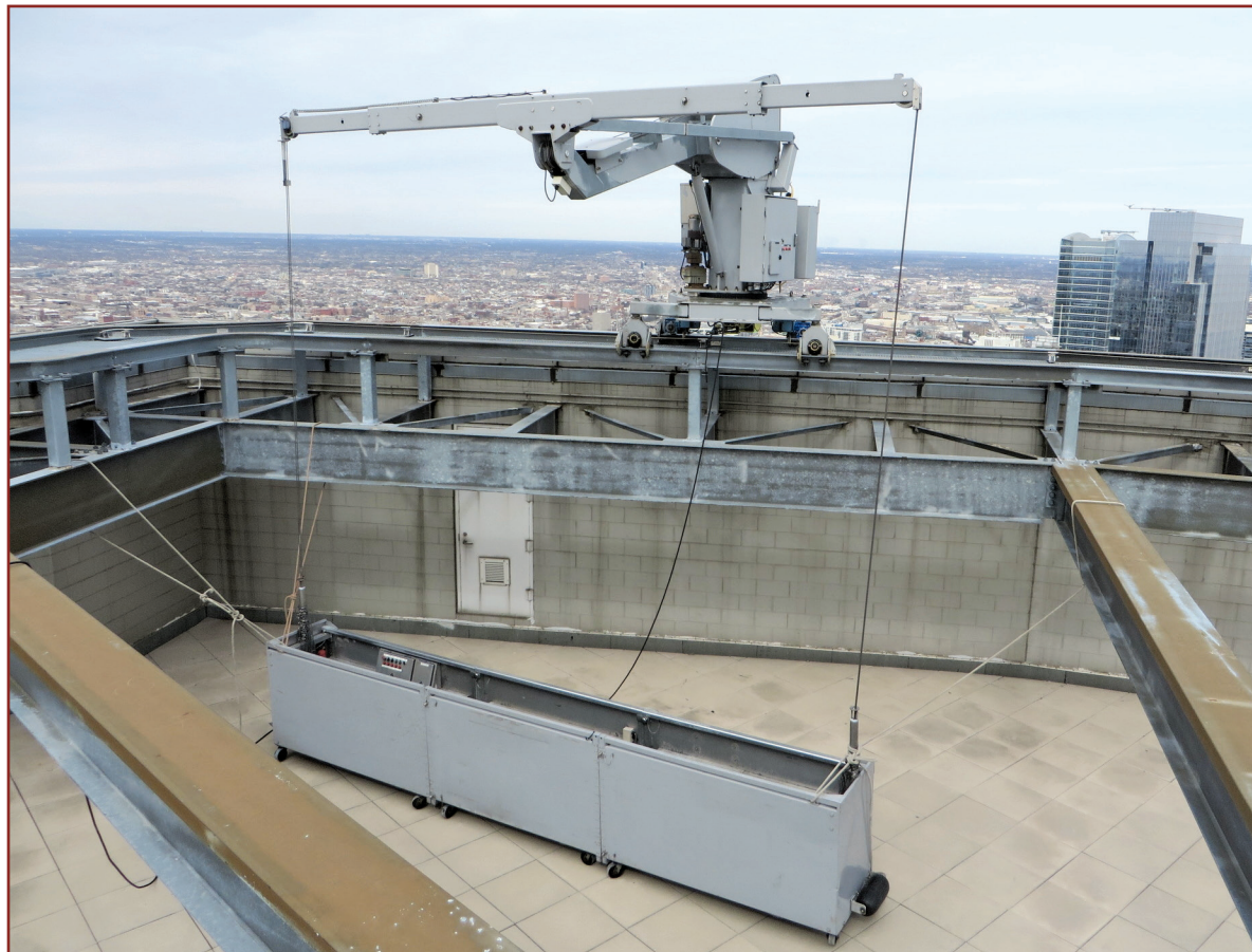
Figure 1 – Large, rail-mounted rooftop carriage.
