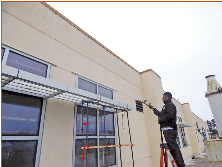
Photo 8 – AAMA nozzle testing at the upper right corner (see Photo 9 ) of this window produced interior leakage at the sill.
