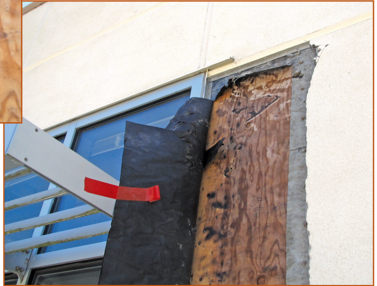
Photo 12 – We continued to trace the water trail up the wall toward the window head.
