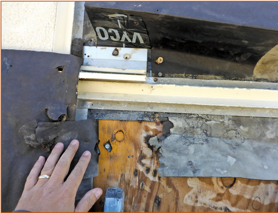
Photo 15 – The trail of water damage leads directly to the head flashing and J-mold accessory above the horizontal reveal.
