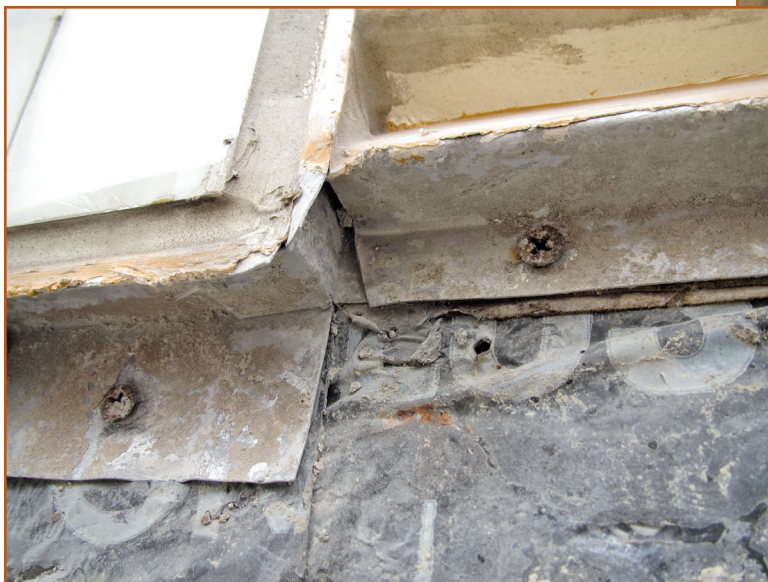
Photo 2 – Bugle-head “self-drilling tapping screws” were used to secure the stucco accessories and trim to the underlying plywood sheathing and wood framing.
