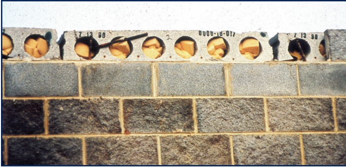
Figure 3 – Hollow-core planks are a form of “pre-stressed” concrete. That is, they have embedded tendons consisting of either steel rods or cables of multiple strands.
