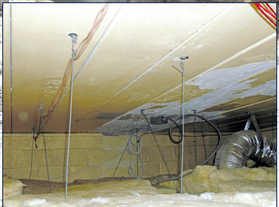
Figure 7 – Hollow-core decks are usually left exposed on the underside, although various inside finishes may be encountered, such as spray-on textures. Suspended ceilings will require some type of attachment for the grid. These deck units are best left without drill holes, as fastening difficulties can arise.
