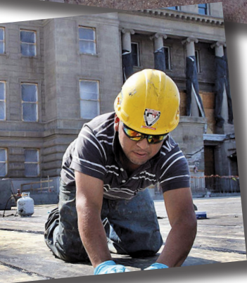
Figure 5 – Waterproofing system application.
