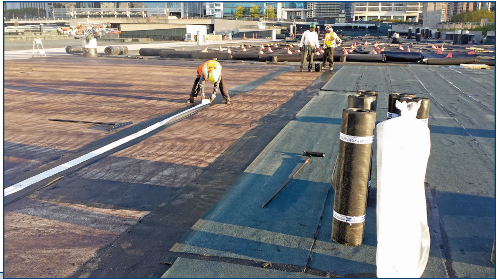
Figures 5-7 – Crews used hot-applied rubberized asphalt to waterproof the parking garage beneath Maggie Daley Park in downtown Chicago, IL. The project required seven layers, including over 1.3 million pounds of rubberized asphalt.
