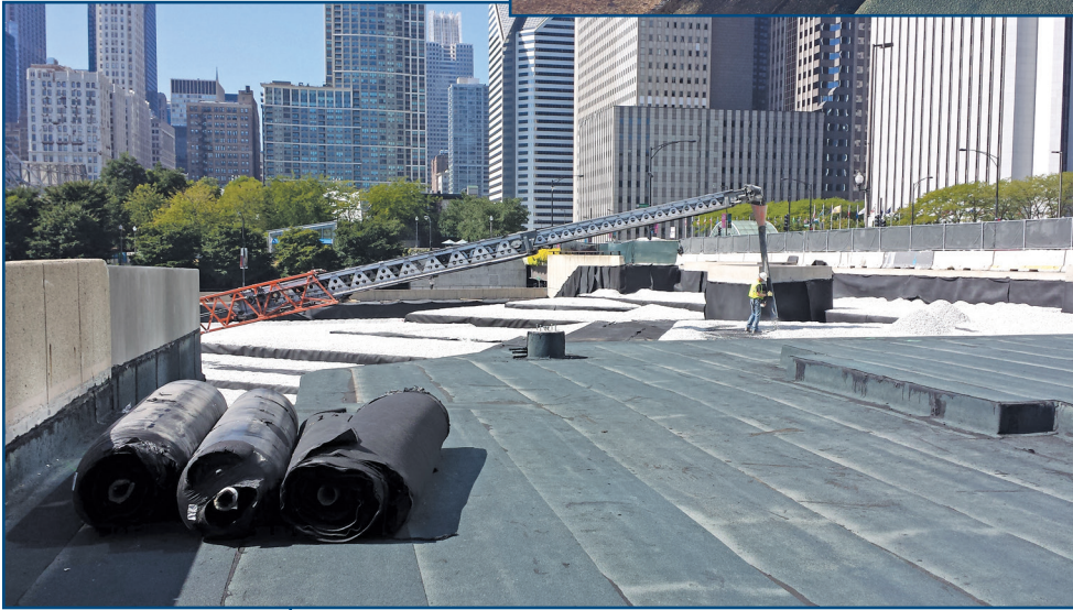
Figures 5-7 – Crews used hot-applied rubberized asphalt to waterproof the parking garage beneath Maggie Daley Park in downtown Chicago, IL. The project required seven layers, including over 1.3 million pounds of rubberized asphalt.
