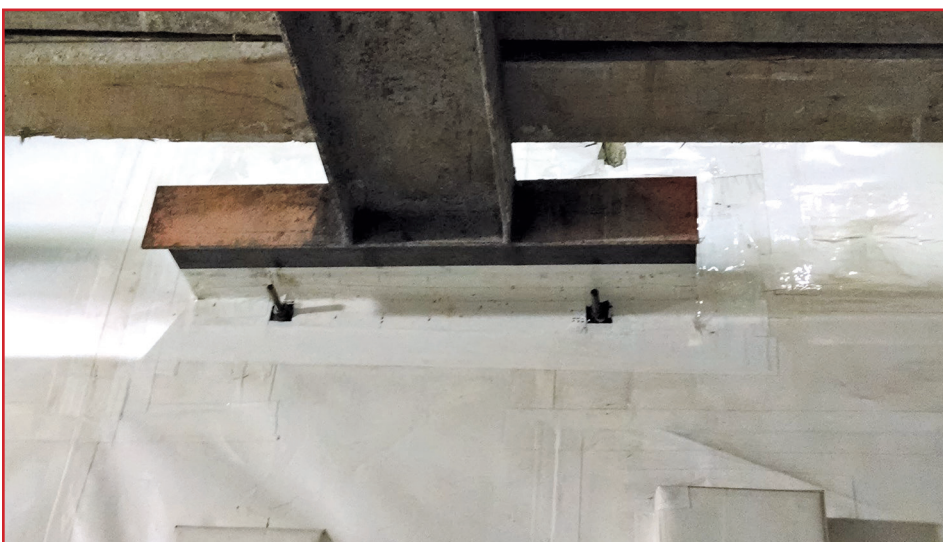
Figure 9 – Waterproofing is being flashed to a waler brace.
