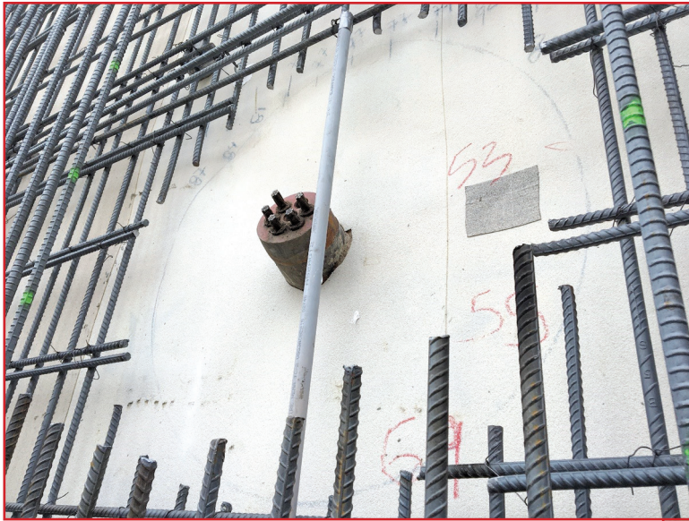
Figure 5 – Tie-back waiting to be waterproofed.
