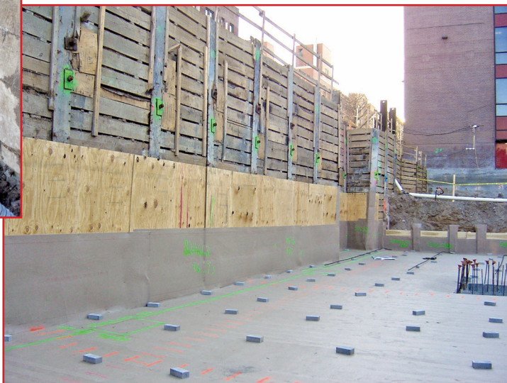
Figure 2 – Plywood utilized to provide smooth substrate for the blindside waterproofing.
