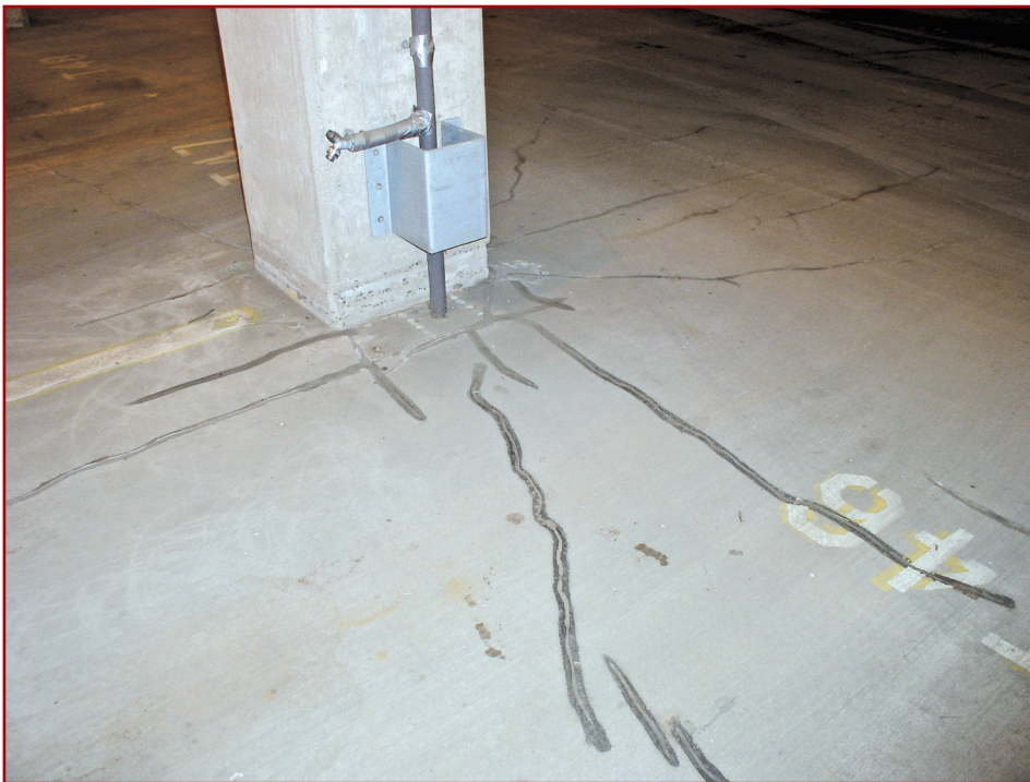
Figure 2 – Cracks are routed and sealed before application of a penetrating sealer.
