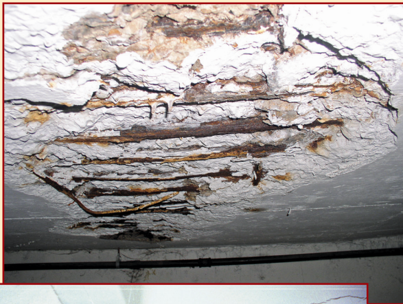
Severe concrete deterioration at the coated underside of a parking deck.
