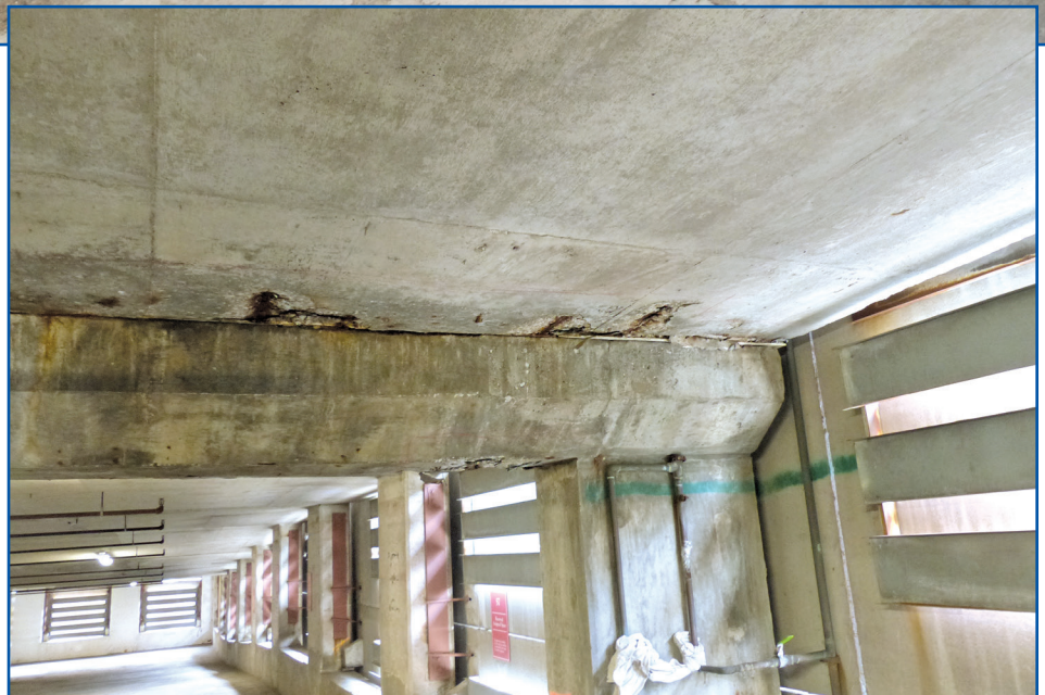
Figure 2 – Corrosion of reinforcing steel.
