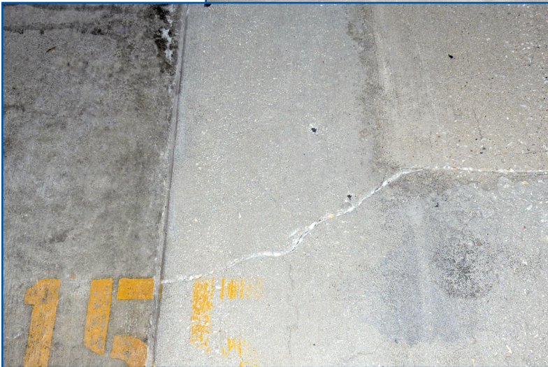
Figure 12 – Shotblasted surface.
