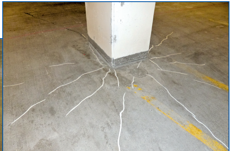
Figure 14 – Routed and sealed cracks.
