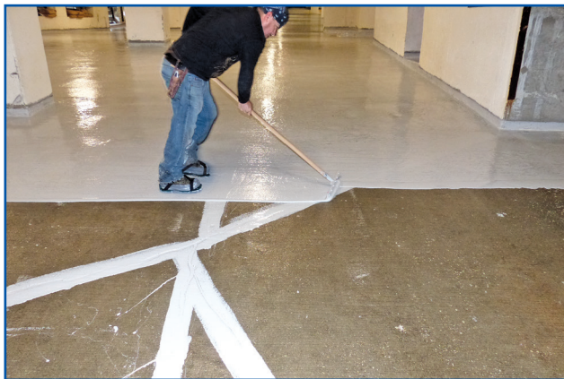
Figure 19 – Base coat application.
