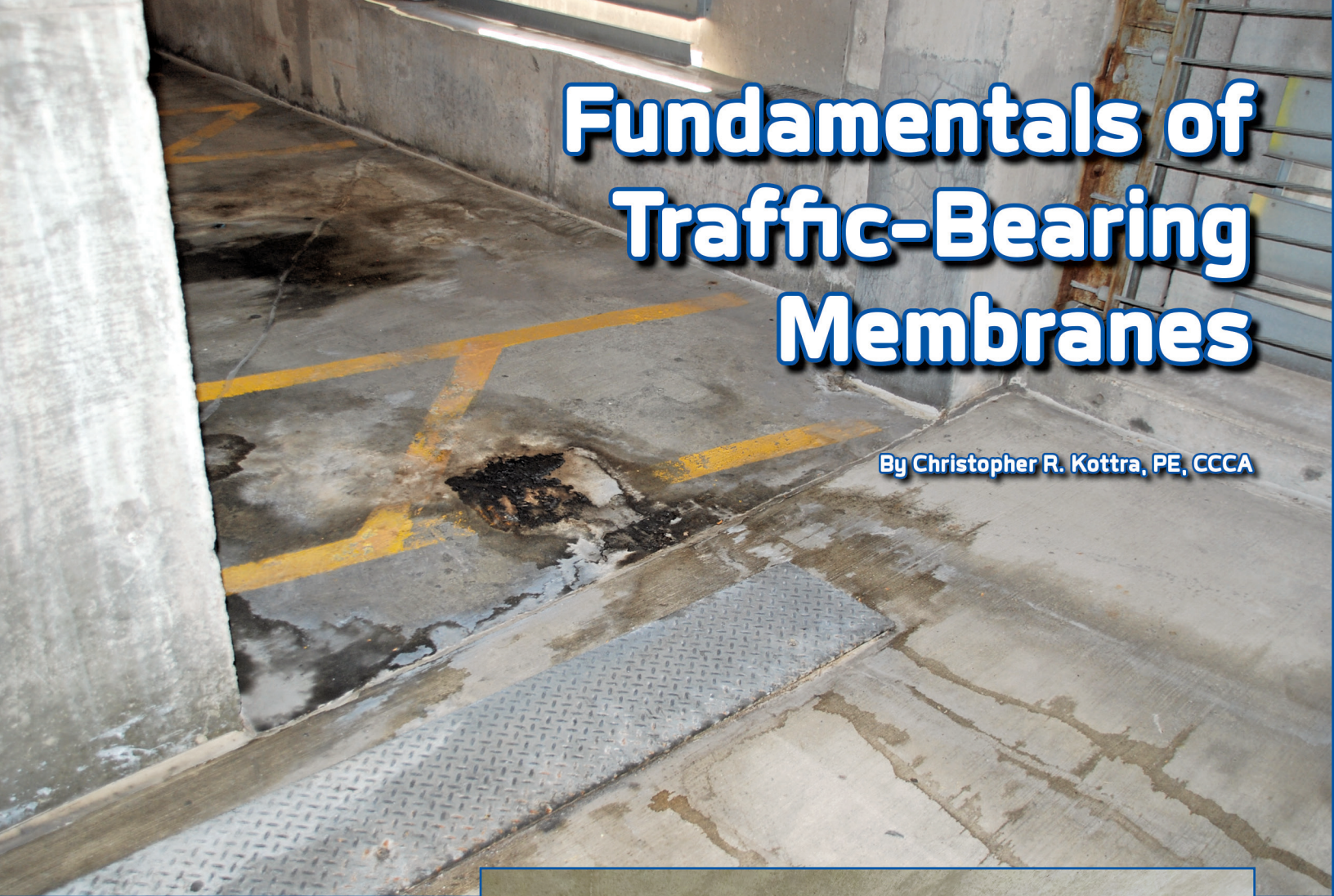
Figure 1 – Chloride exposure.
