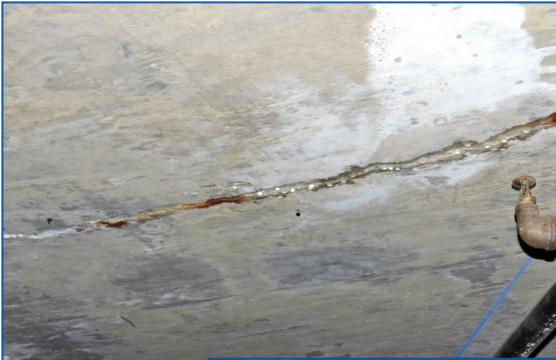
Figure 3 – Moisture migration through slab.
