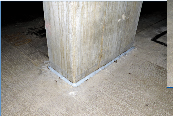
Figure 15 – Sealant at horizontal-to-vertical transitions.
