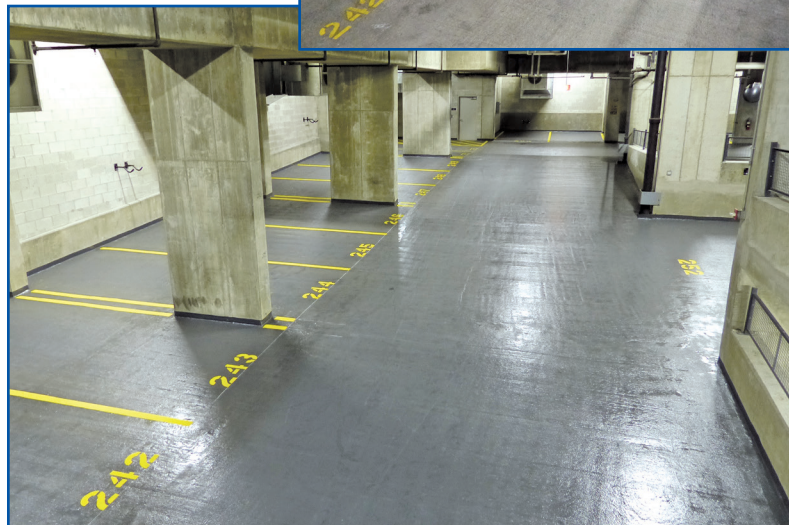
Figure 6 – Parking garage slab after TBM application.
