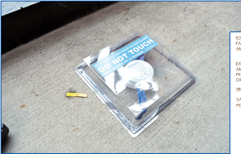
Figure 7 – ASTM F1869 moisture emission testing.
