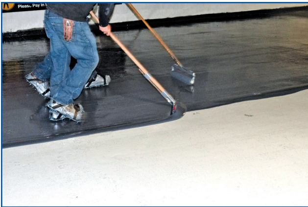
Figure 20 – Intermediate coat application.
