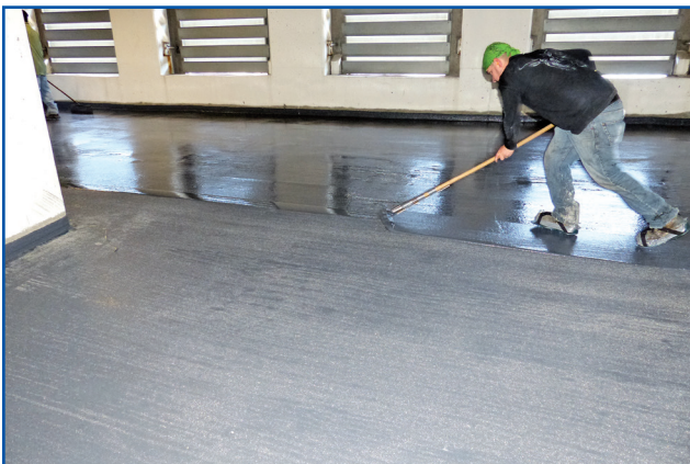
Figure 22 – Finish coat application.
