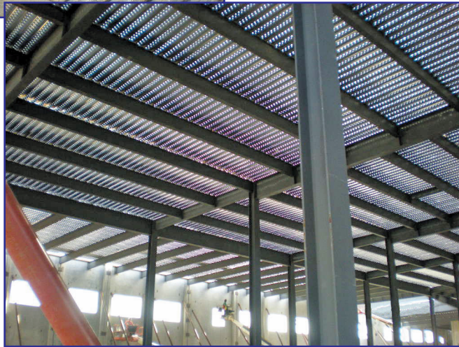
Figure 2 – Metal pan deck construction.
