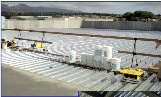
Figure 1 – Metal pan deck construction.
