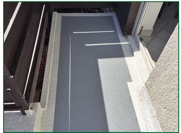
Figure 3 – PMMA balcony coating application with two-tone aesthetic (courtesy Soprema).
