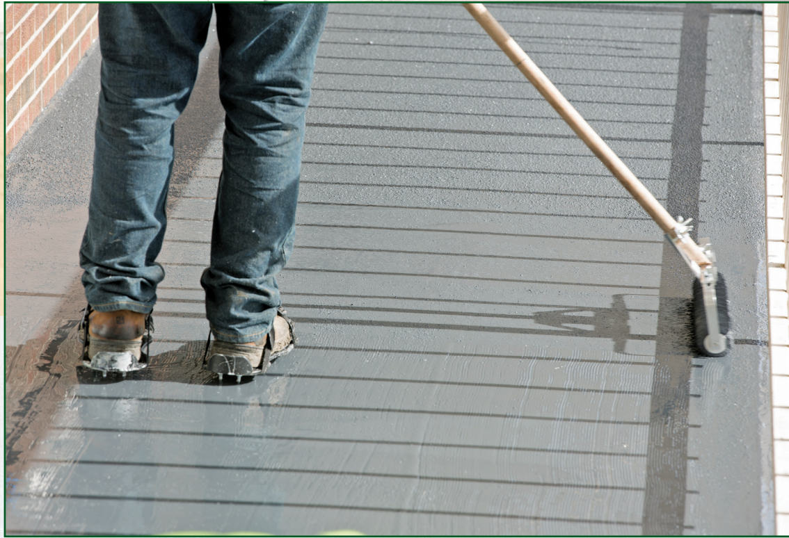
Figure 1 – Liquid urethane coating application in progress (courtesy BASF).
