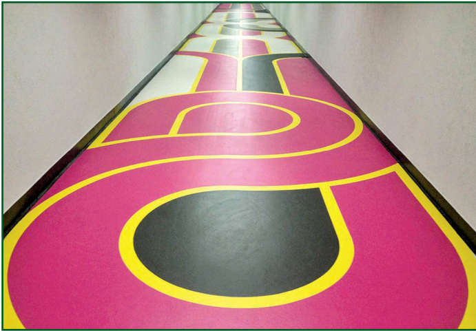
Figure 4 – PMMA hallway coating with multicolored finish pattern (courtesy Soprema).
