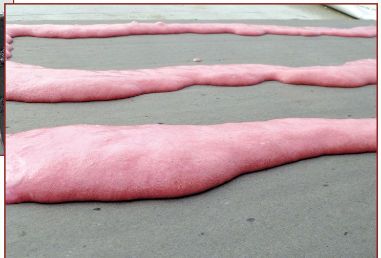
Figure 2 – Liquid beads of adhesive spread to several inches wide and rise \frac{3}{4} to 1 inch above the substrate.
