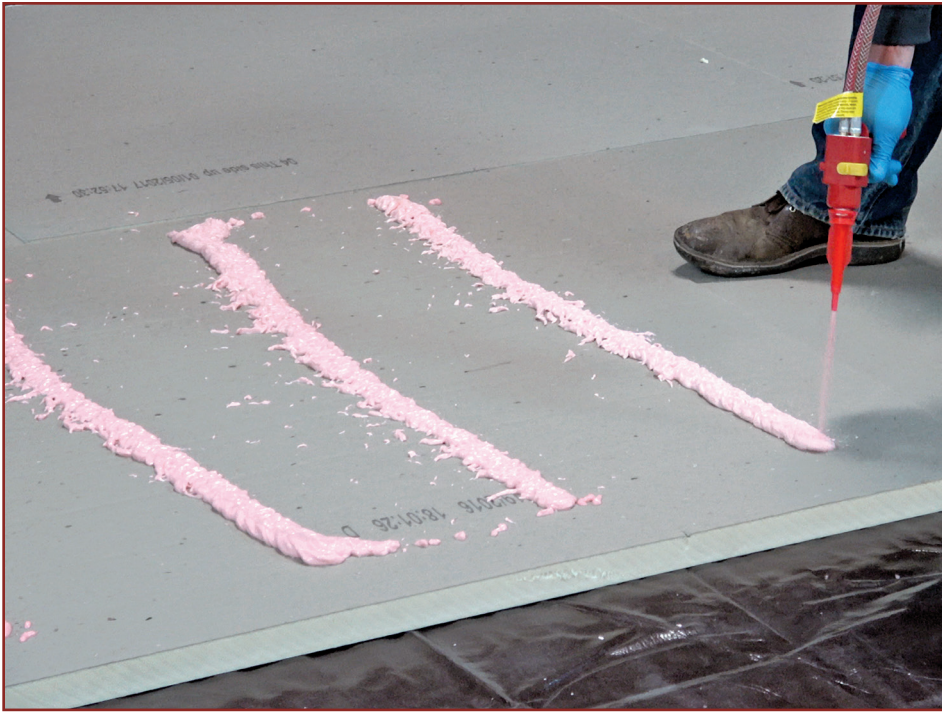
Figure 6 – Some canister adhesives can yield up to 40 or more squares of coverage per set using the “parallel line” application method.
