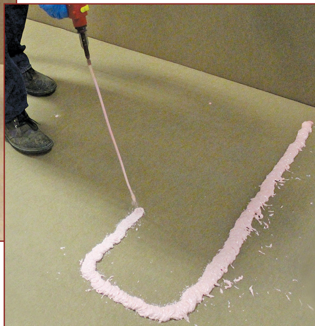
Figures 4 and 5 – The most common application is a continuous serpentine bead at the prescribed bead spacing—typically 12 inches on center.
