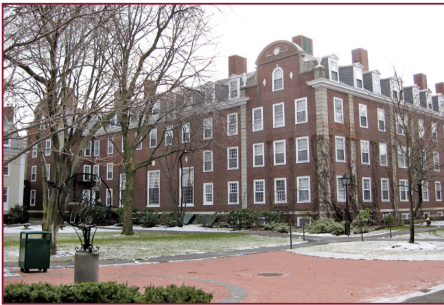
Figure 1 – Typical solid masonry wall dormitory.
