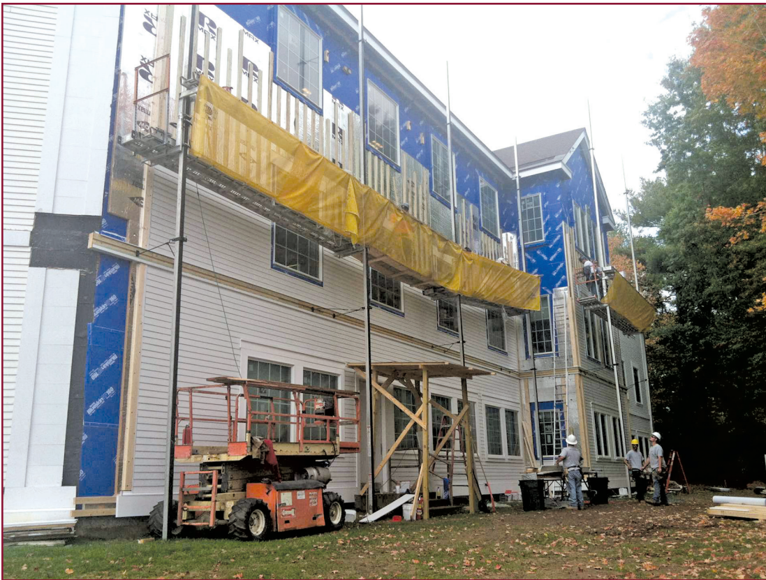
Figure 22 – Exterior wall assembly under construction.
