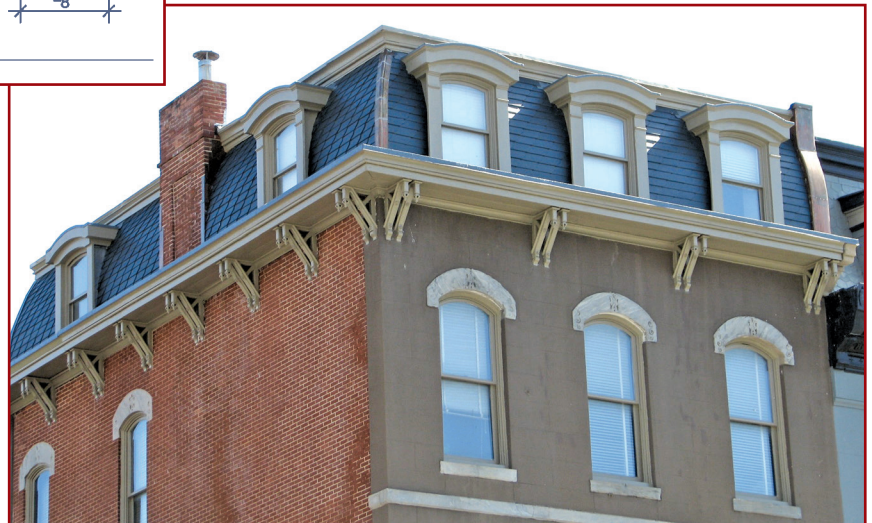
Figure 12 – View of new right-handed Dutch Lap slates at the mansion.
