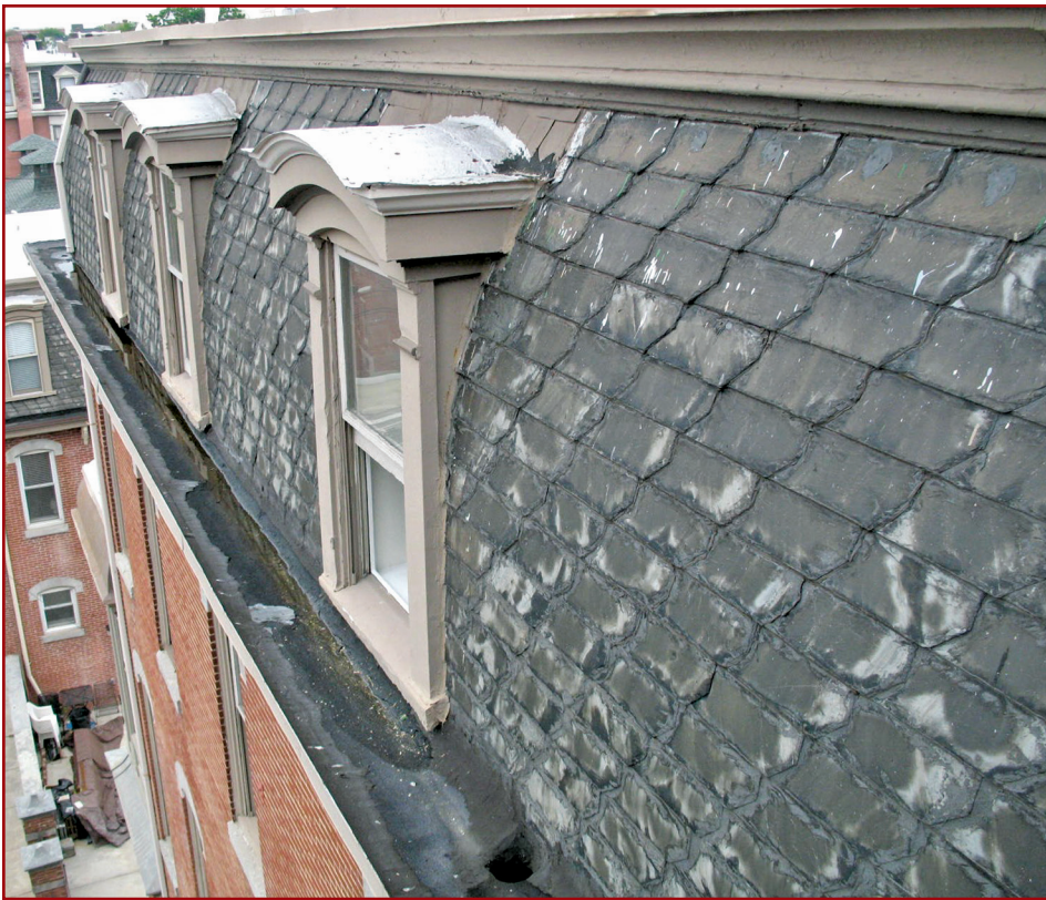
Figure 2 – Original Dutch Lap slates on the mansion’s convex mansard roof.
