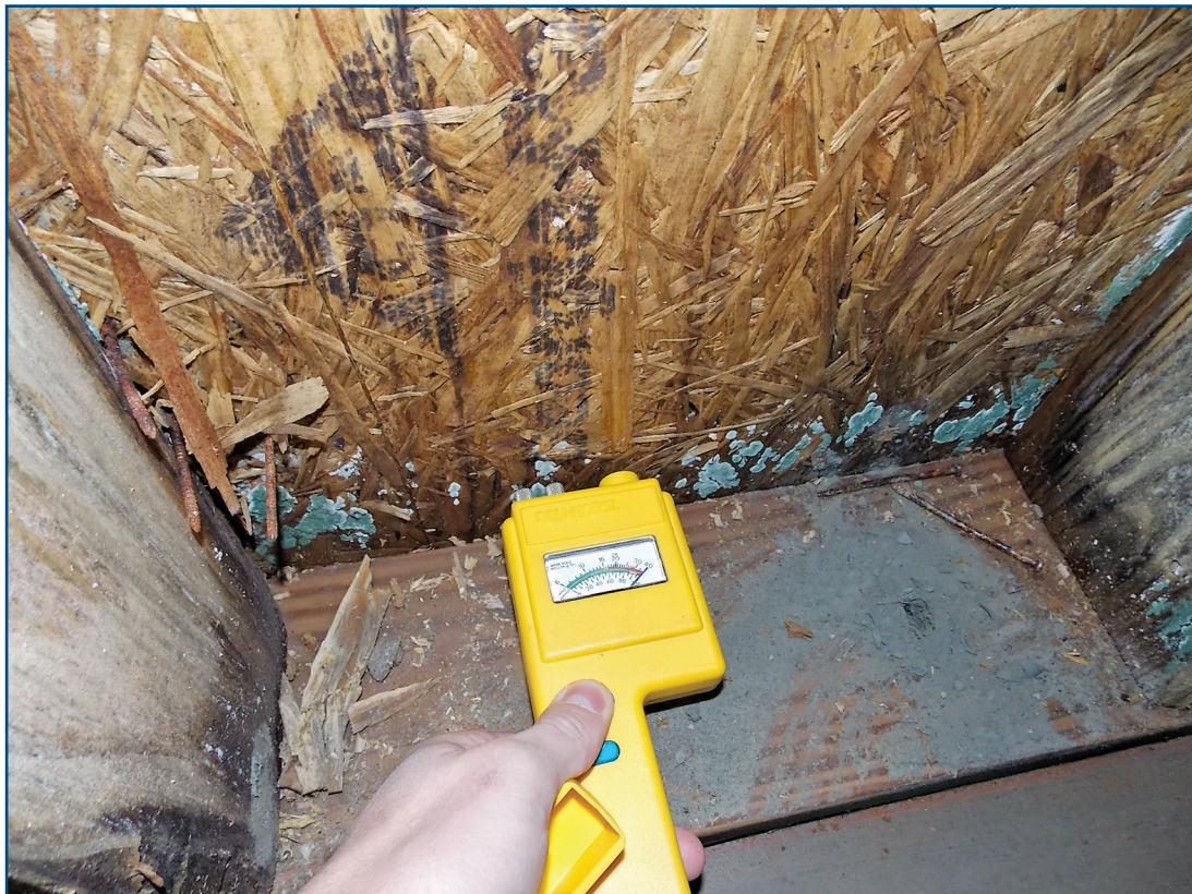
Figure 6 – Water intrusion/damage of a mid-rise wood frame building under construction.
