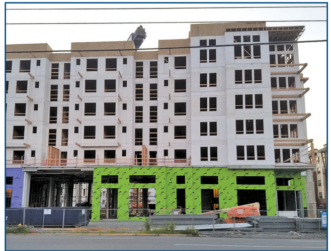
Figure 1 – Typical mid-rise wood frame building under construction.
