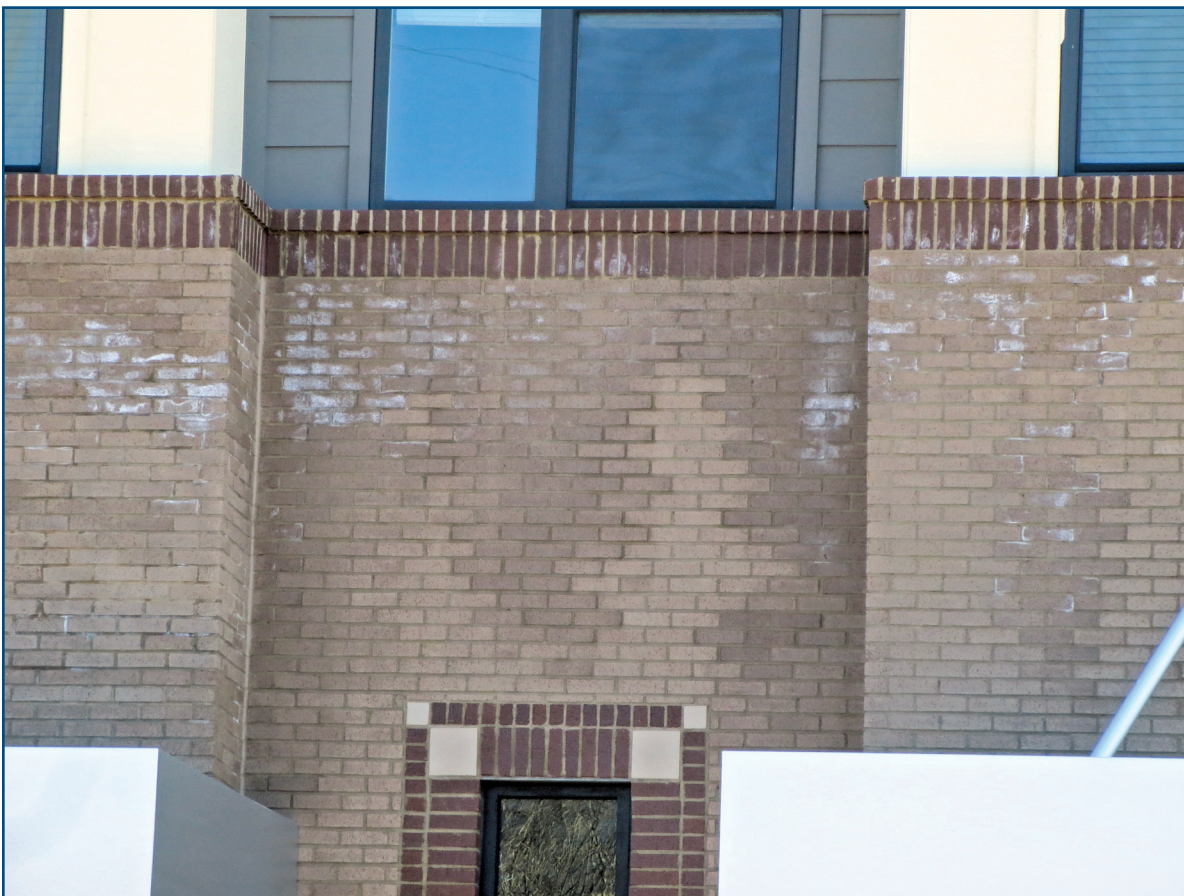
Figure 2 – Wall modulation with efflorescence.
