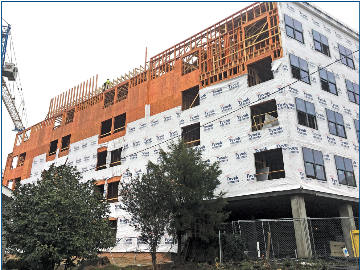
Figure 7 – A haphazard sequencing of multiple trades on the exterior wall of a building under construction.
