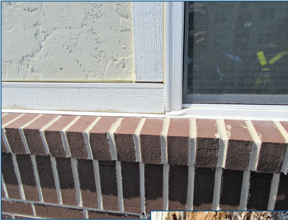
Figure 3 – Window damage caused by differential building movement.
