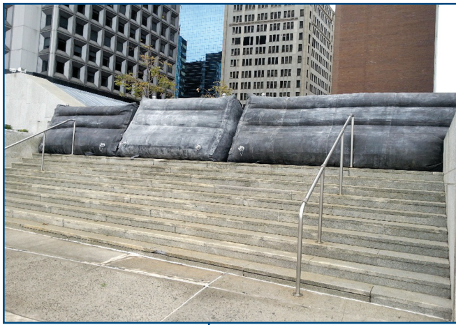
Figure 5 – Flood balloons installed as part of a training drill.
