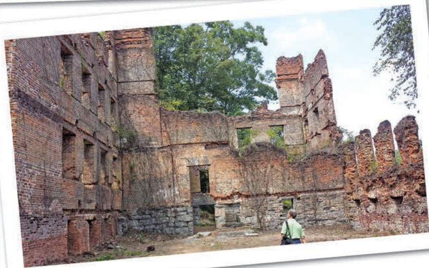
Photo 3 – View of mill interior before repair.
