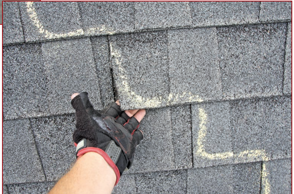
Figure 5 – Unbonded diagonal pattern of shingle overlaps.
