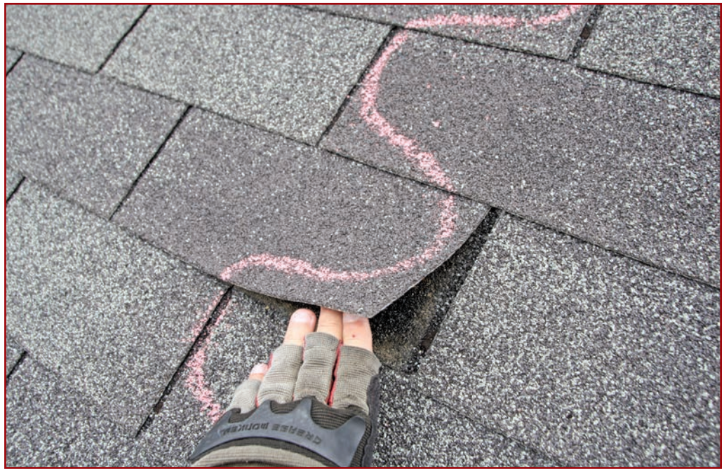
Figure 6 – Unbonded racked pattern of shingle overlaps.
