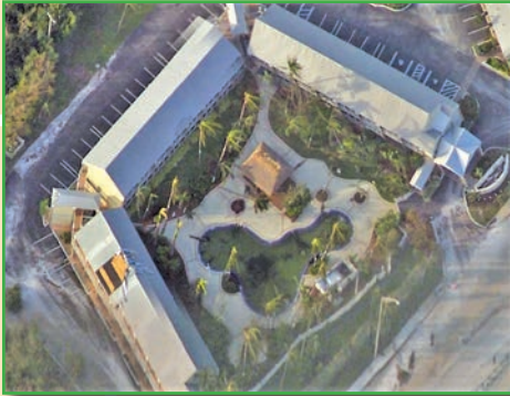
Visible damage to less than 10% of these hotel roofs.
