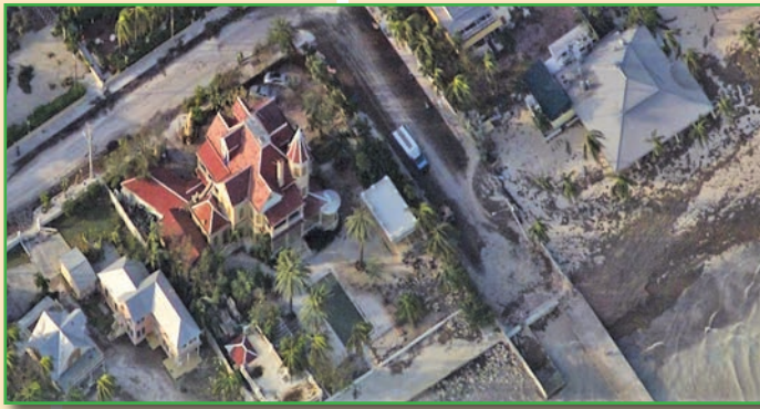
No conspicuous roof damage to the various roofs covering these Key West residential structures.
