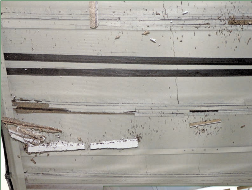
Figure 9 – Spalled concrete caught in netting with exposed unpainted concrete and reinforcing steel.
