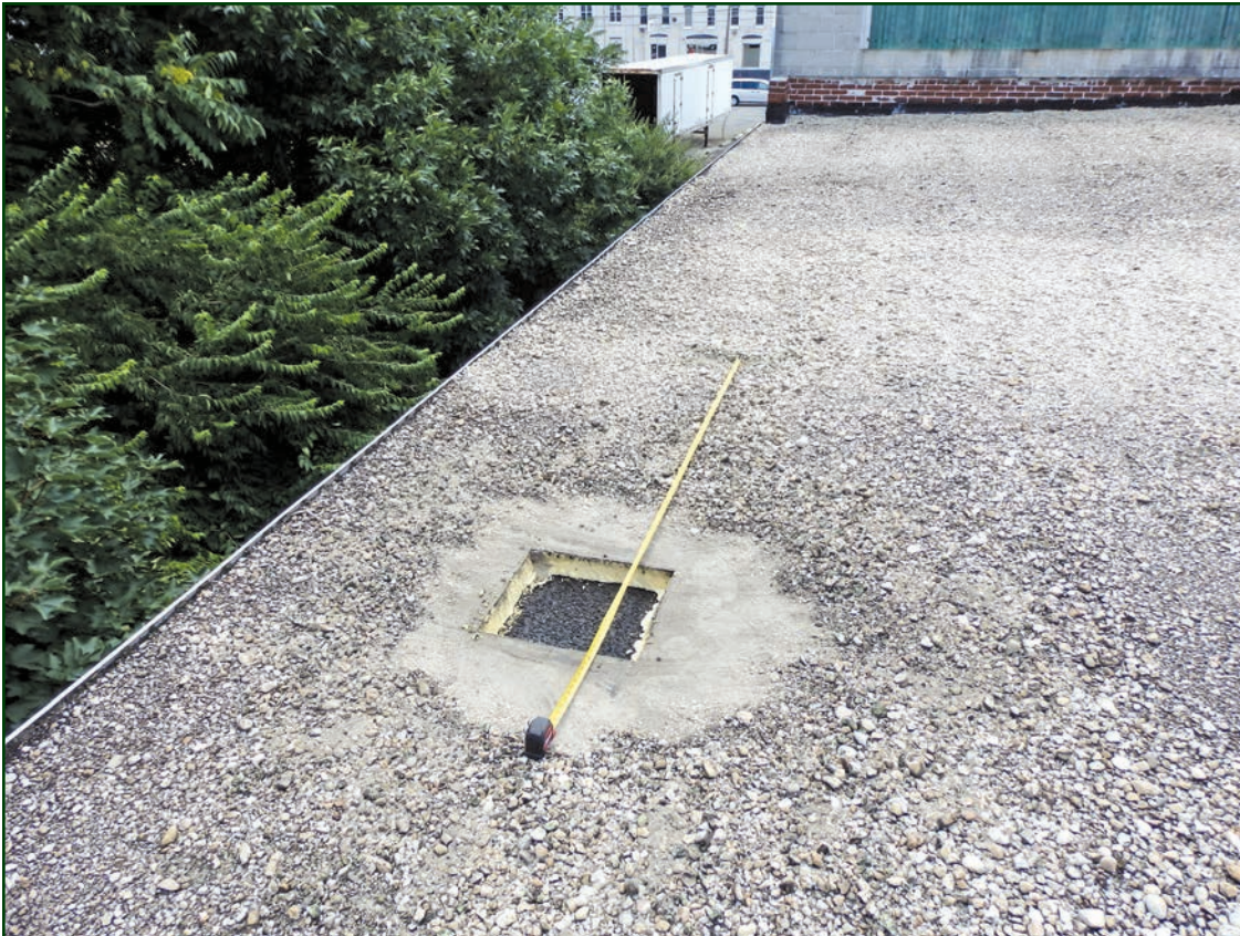
Figure 6 – Overview of roof assembly at low-bay area.
