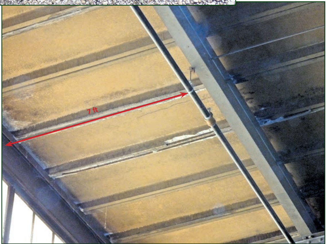
Figure 7 – Precast concrete channel slab planks at the roof deck.
