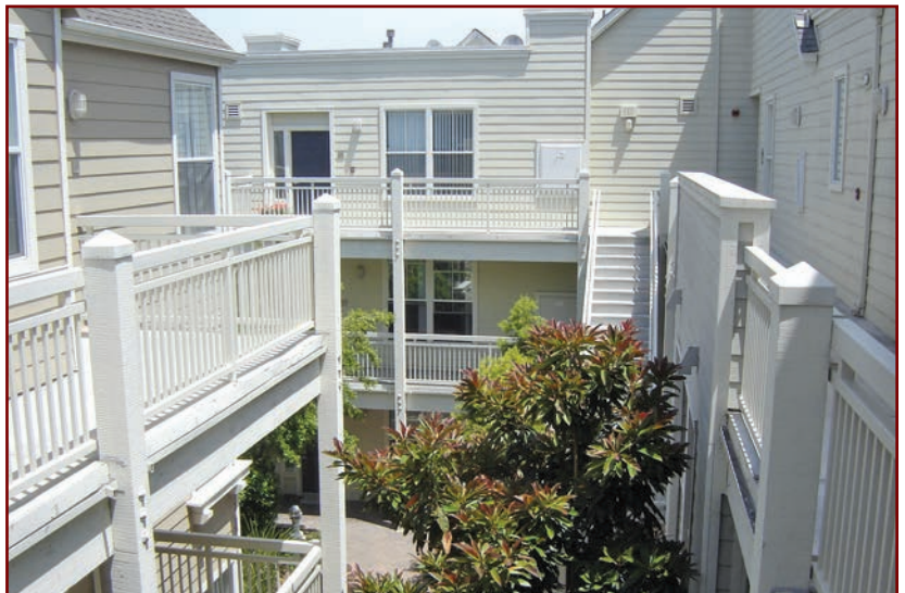
Figure 1 – Upper-story tenants at this apartment complex are served by 3000 lineal feet of wood-framed elevated walkways.
