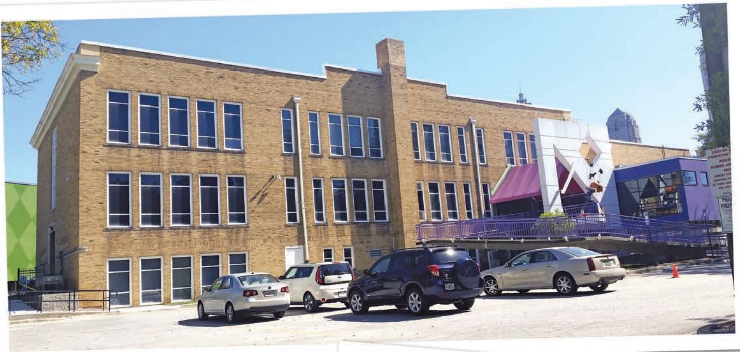
Figure 2 – Overall view of west elevation.
