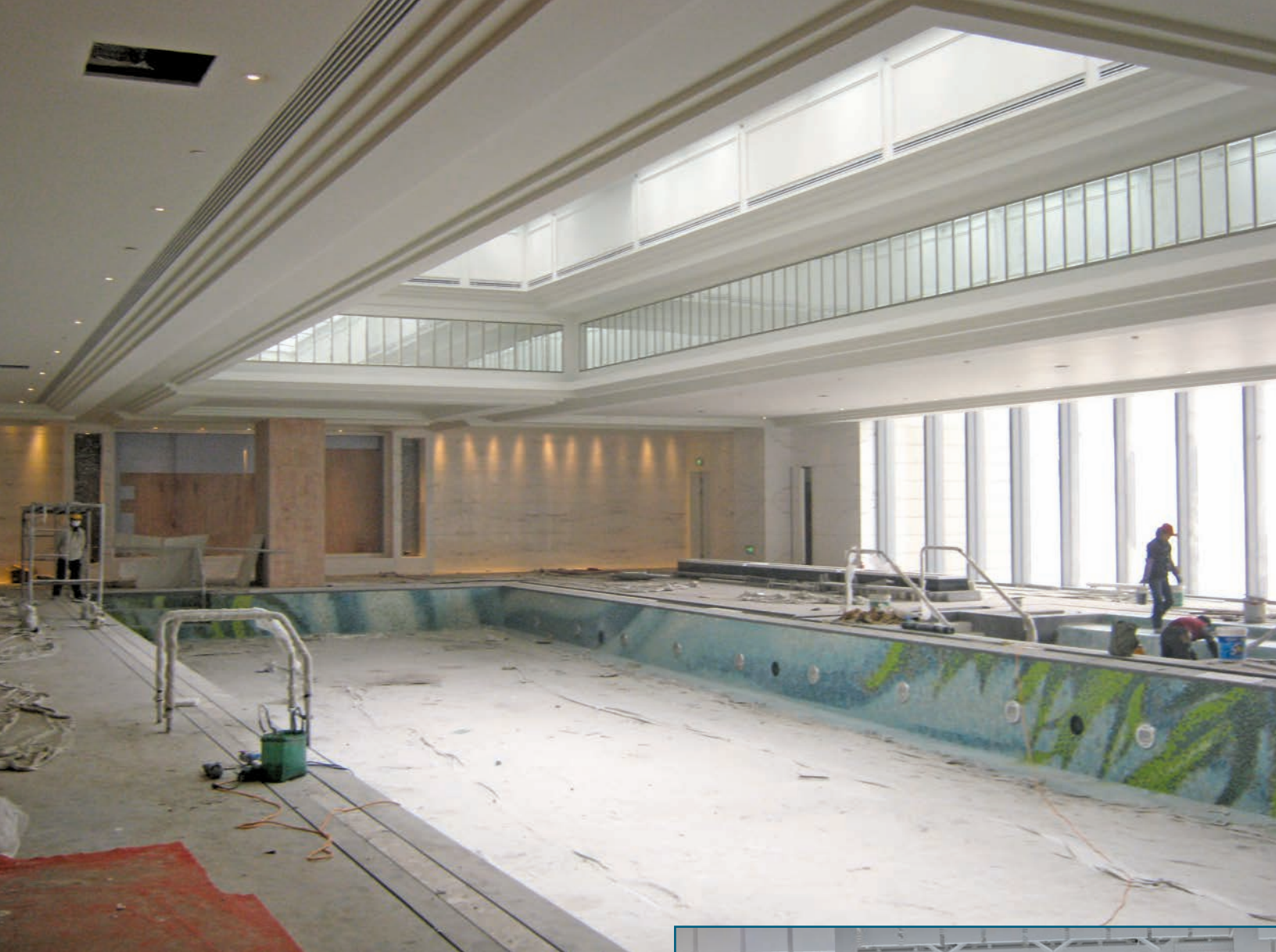
Figure 2 – Four Seasons Tianjin. © WSP.
