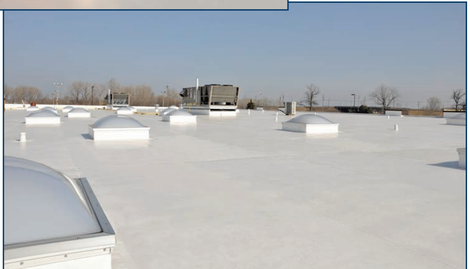
Figure 3 – Custom prefabricated curb flashings.
