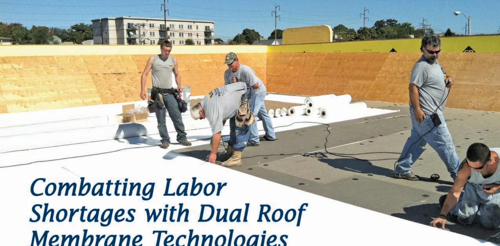
Figure 1 – Typical thermoplastic roofing job site and crew.
