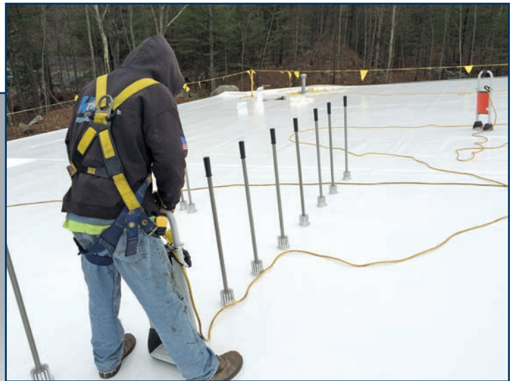
Figure 9 – Induction welding production process.
