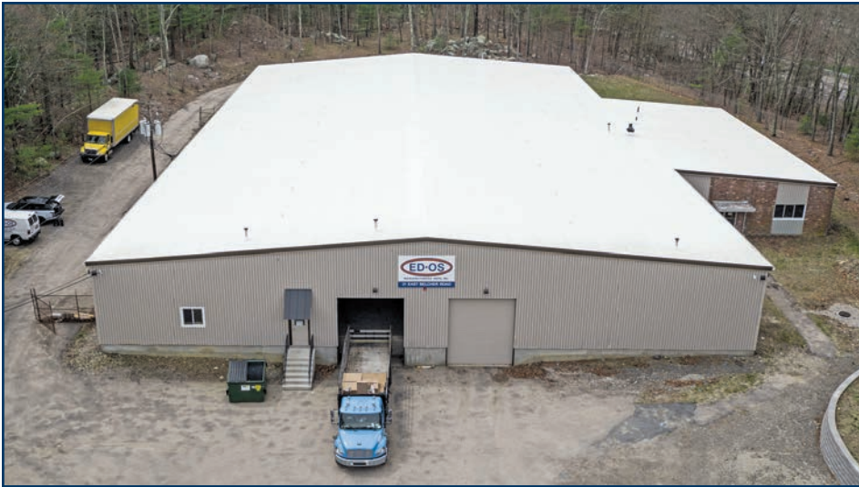
Figure 10 – Metal roof recovery combining purlin fastening and induction welding.
