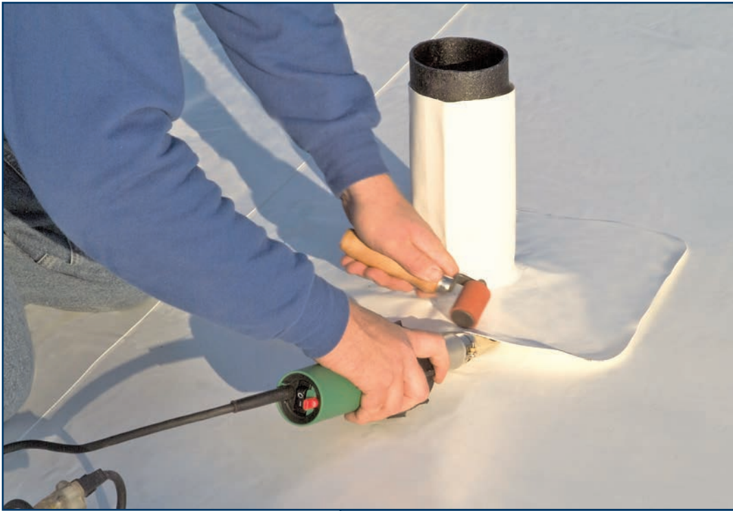
Figure 2 – Prefabricated pipe stack flashing.
