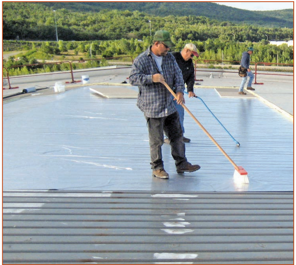
Figure 6 – Air barrier being installed directly to a metal deck.
