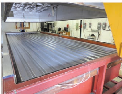
Steel deck installation
