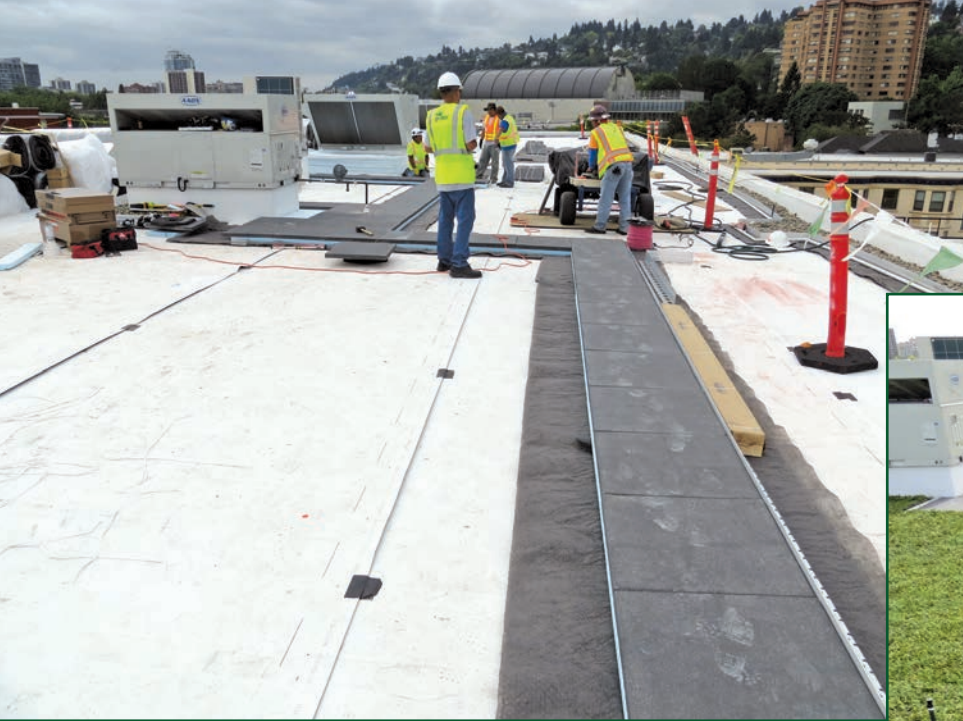
Figures 3 and 4 – Paver path under construction (left) and after planting is complete (below). Photos and diagrams courtesy of DiademUSA.
