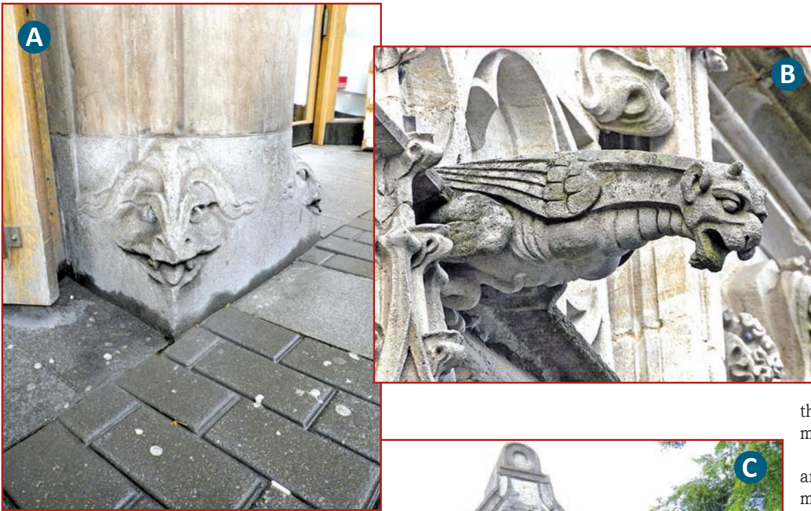
Figure 12 – Photos show the use of granite at the base of a column at a limestone-clad building (12A), and the use of more dense stone material for the gargoyle scupper (12B) as compared with the stone on the building façade. Figure 12C shows a view of a gabled parapet with use of more durable Indiana limestone at the high-exposure regions, including copings and finials, as compared with the rusticated corner quoins constructed of Illinois limestone.
