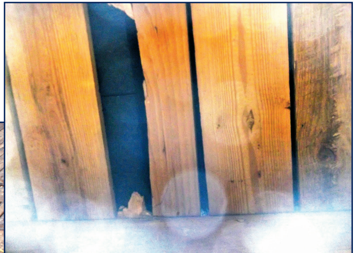
Figure 7 – This newer roof had been installed with little thought given to proper deck repairs.
