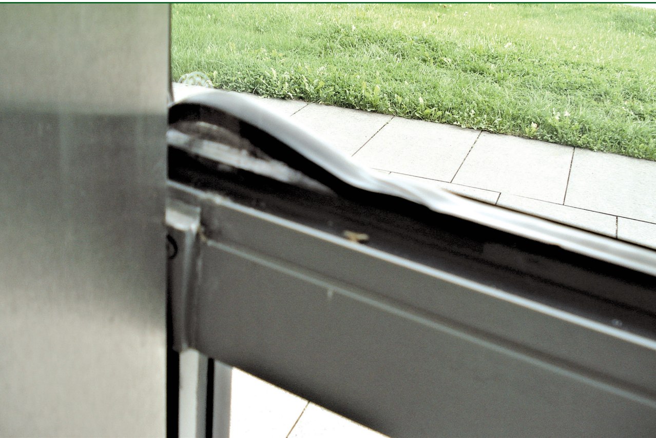
Figure 6 – Example of migration of flexible spacer at IG unit.
