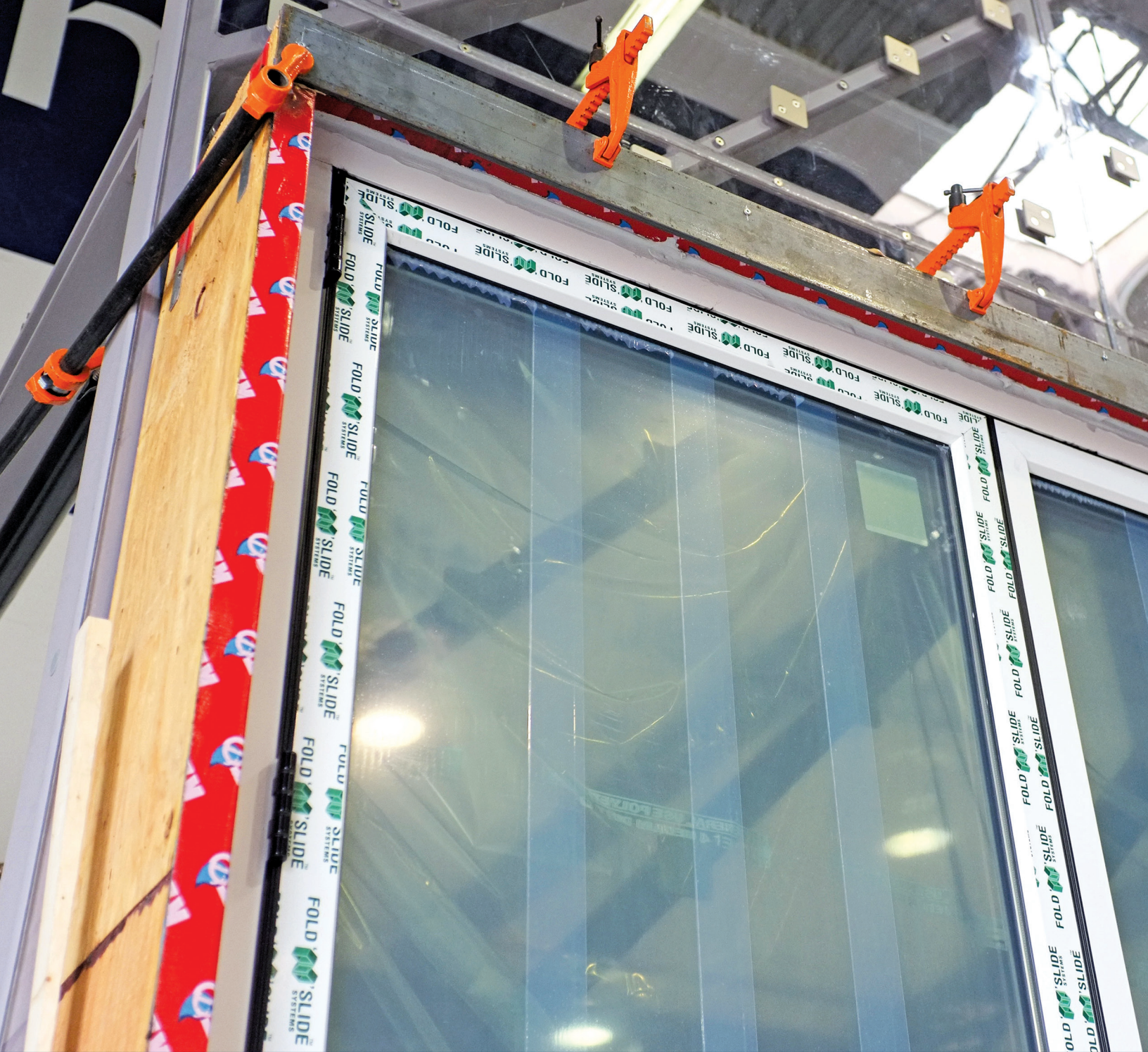
Figure 2 – Close-up of folding door undergoing lab structural testing. Photo by Al Jaugelis.
