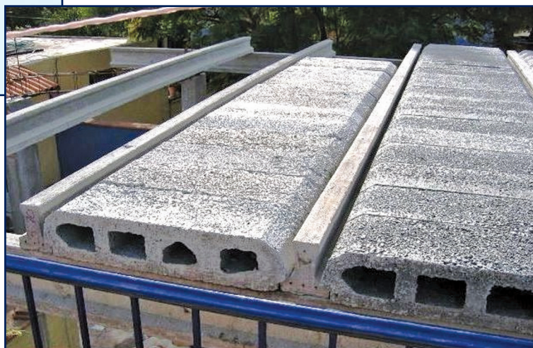
Figure 4 – Note here that the bottom face of hollow-core units is flush with the bottom of inverted T-joists. This was an alternative available to the specifier/designer.
