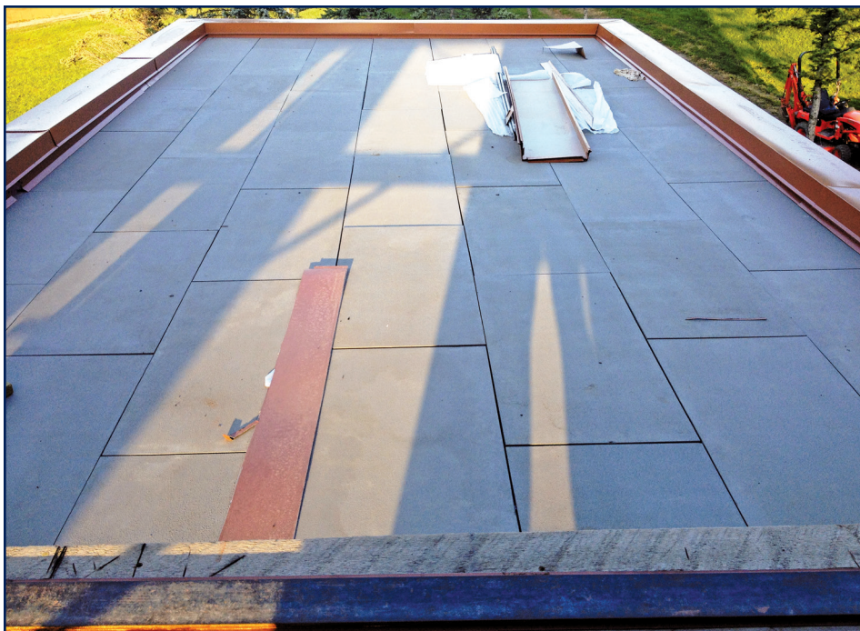
Figure 11 – A nearly finished Supra-Deck, ready for stitching screws. Bituminous roofs were commonly applied to this substrate.
