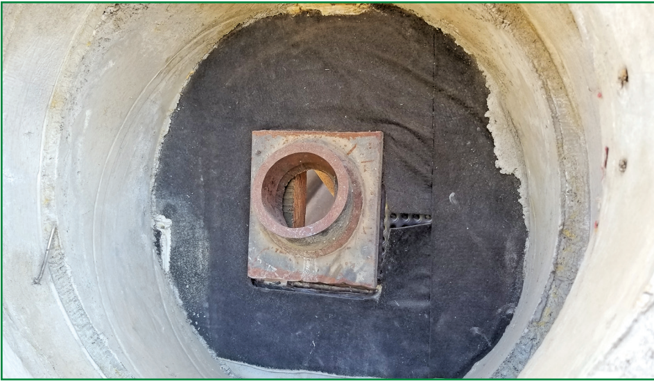
Figure 7 – Earth retention tie-back observed after form work was removed prior to the application of waterproofing detailing.
