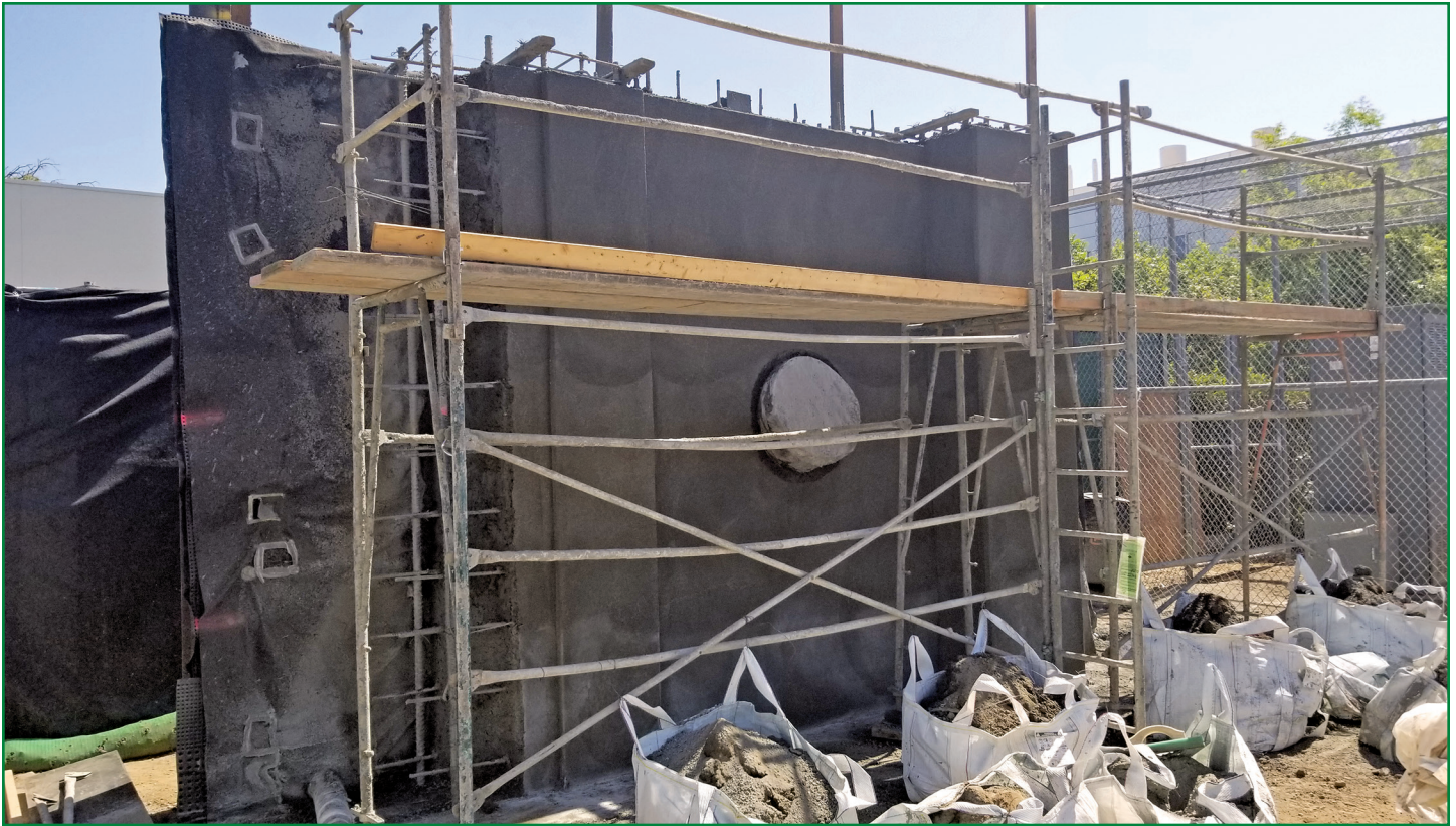
Figure 1 – The stand-alone blindside mock-up shortly after the shotcrete was placed.
