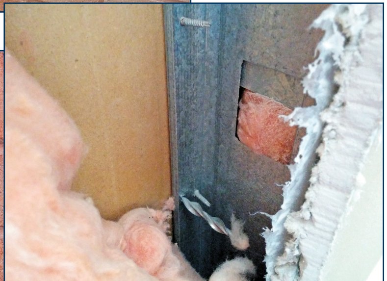
Figure 6 – New retrofit helical brick ties engaged at metal stud backup.
