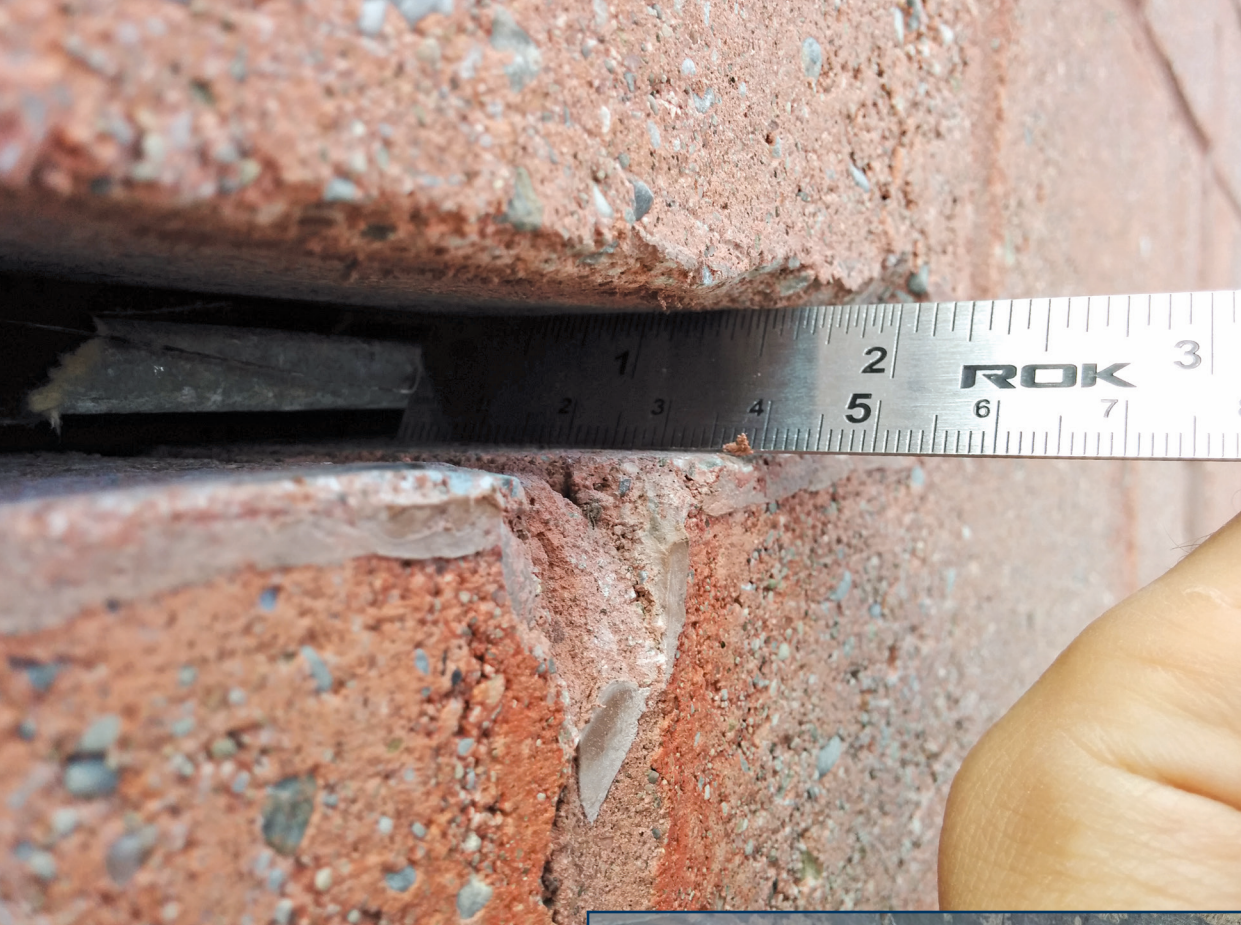
Figure 7 – Checking shelf angle overhang (1¼ in. depicted).
