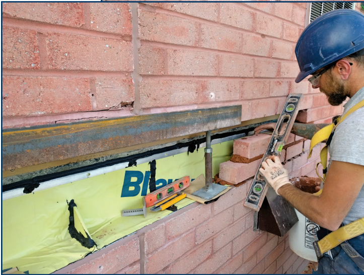
Figure 10 – New through- wall flashing and brick reinstatement.
