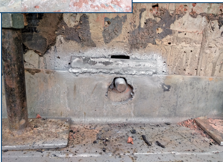
Figure 14 – Repair at cut shelf angle.
