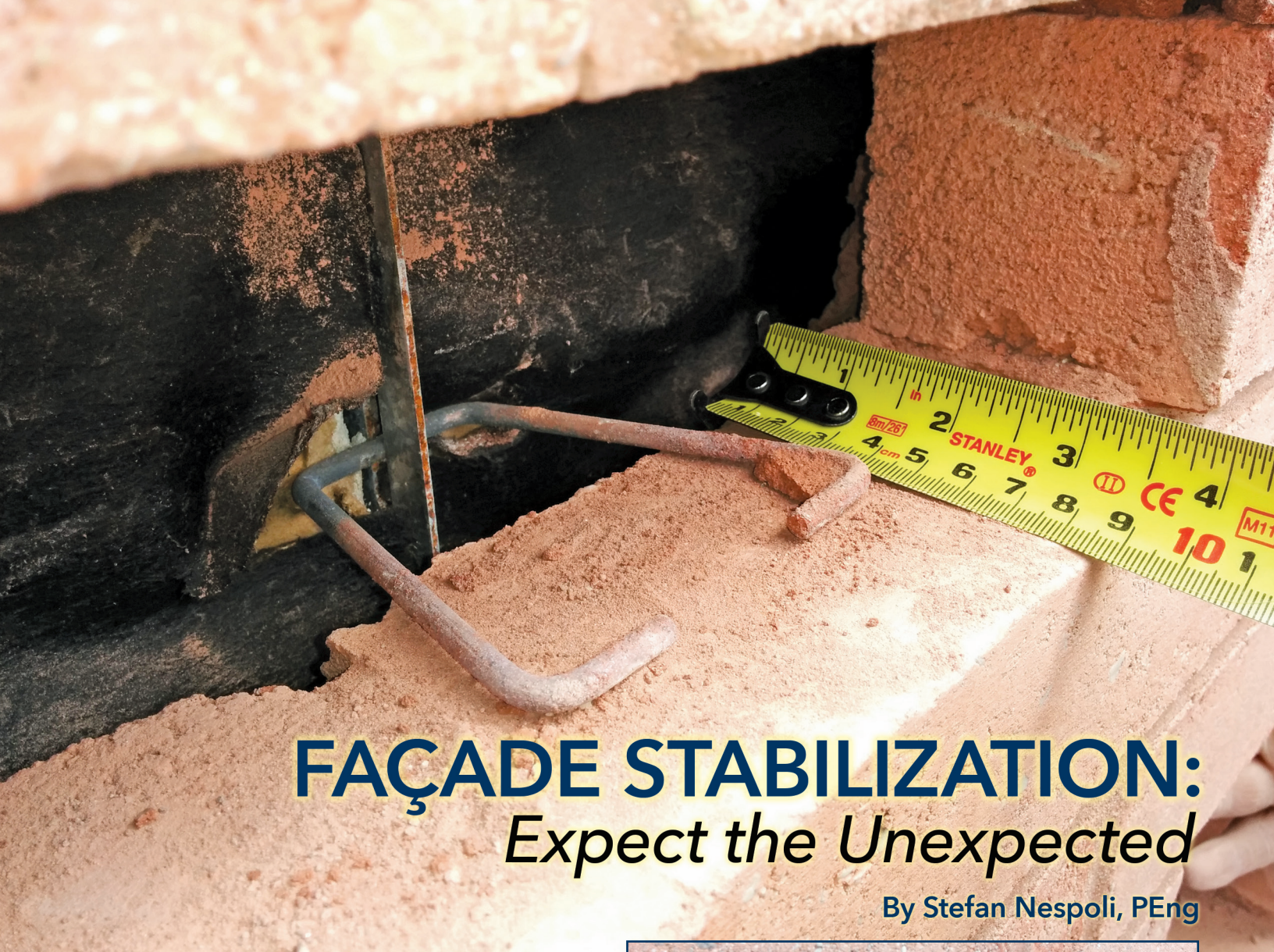
Figure 1 – Correct installation at existing wire-and-plate brick tie at steel stud backup.
