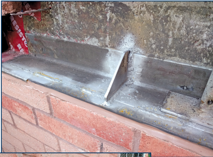
Figure 9 – New shelf angle extension and reinforcing.
