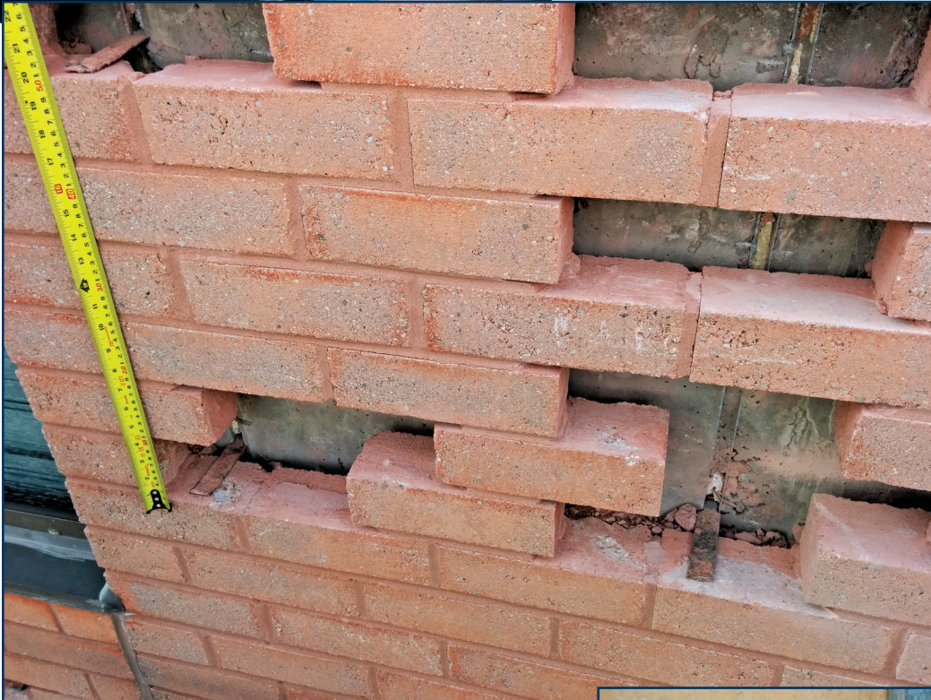
Figure 4 – Existing dovetail brick tie at concrete backup.
