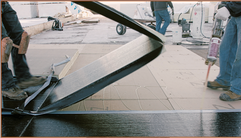
Figure 4 – Use of pre-assembled panels combining roof membrane, cover board, and insulation can accelerate and simplify installation, which can be an advantage when contractor crews are stretched thin. Photo courtesy of Soprema.
