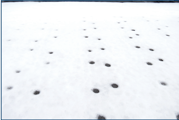
Figure 5 – Thermal bridging on snow-covered roofs from rooftop penetrations and fasteners.
