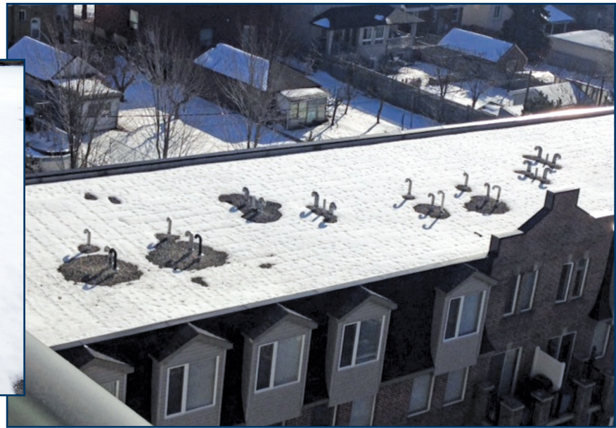
Figure 5 – Thermal bridging on snow-covered roofs from rooftop penetrations and fasteners.
