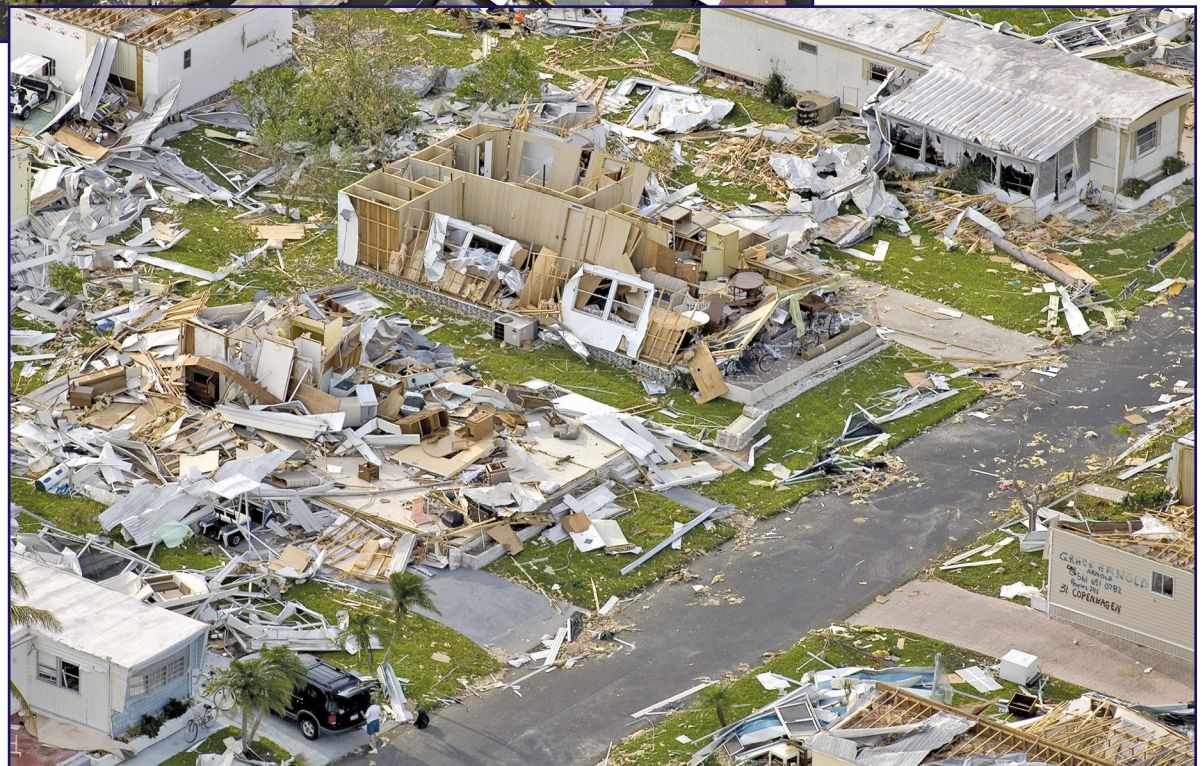
Figure 3 – Hurricane damage to houses. (Image 63005, www.pixabay.com)
