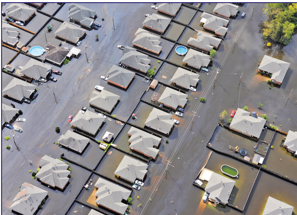
Figure 4 – Flood damage to neighborhood houses. (Image 642586, www.pixabay.com)
