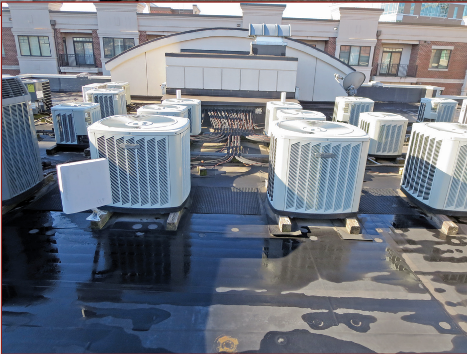
Figure 4 – Dead load from mechanical units.
