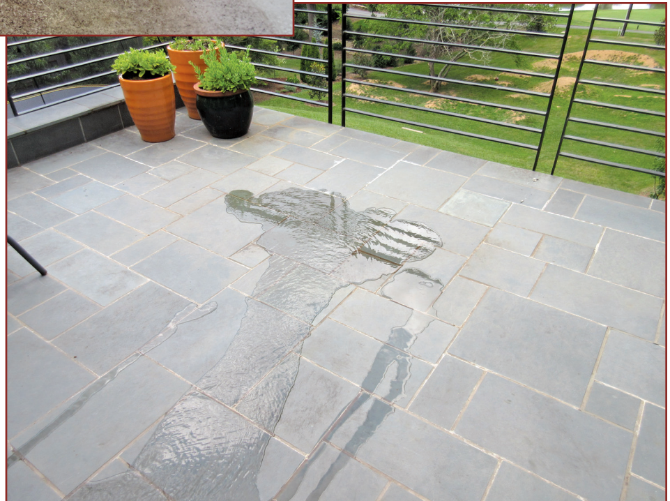
Figure 8 – Balcony ponding.
