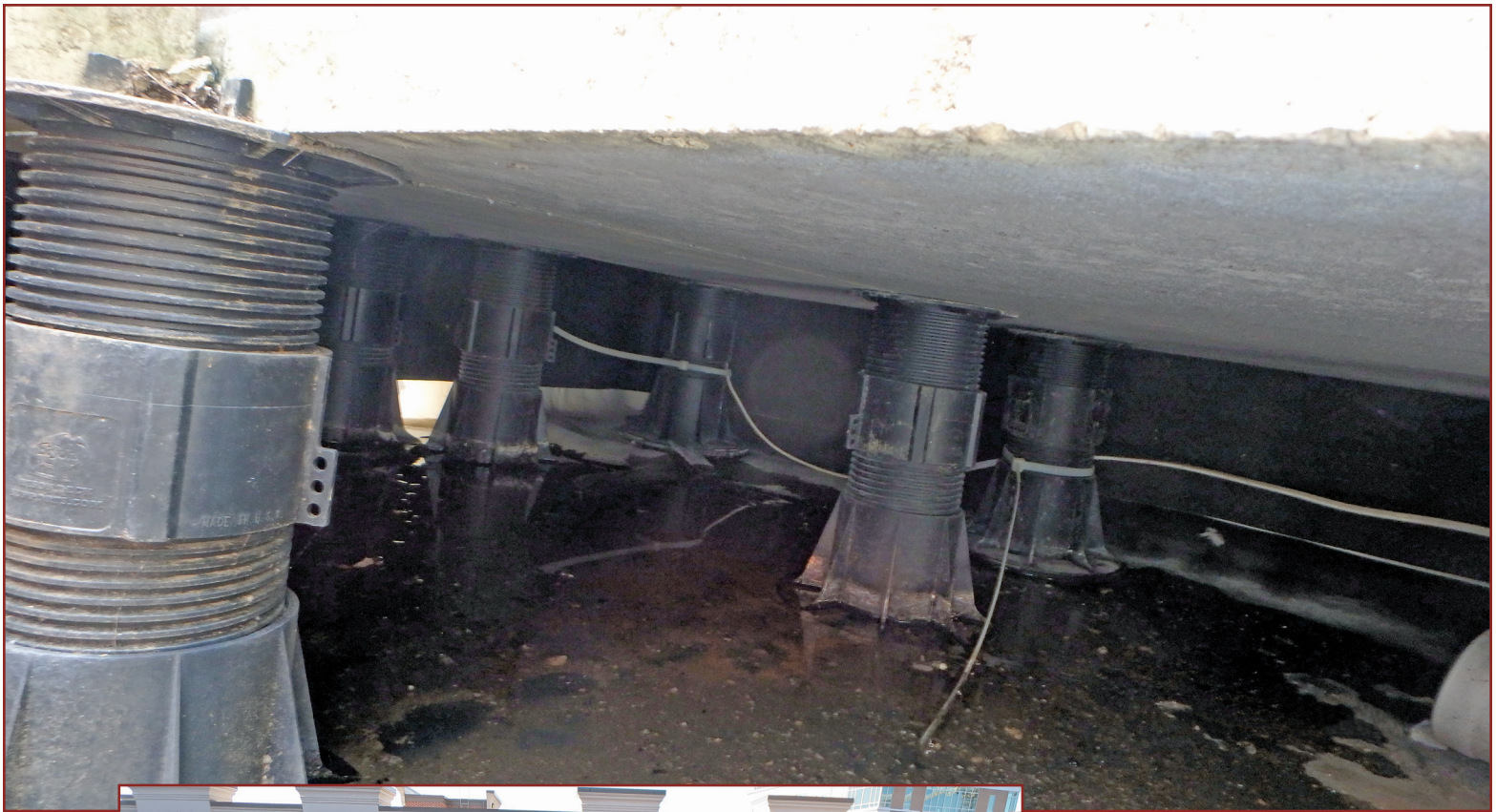
Figure 3 – Dead load from paver system.
