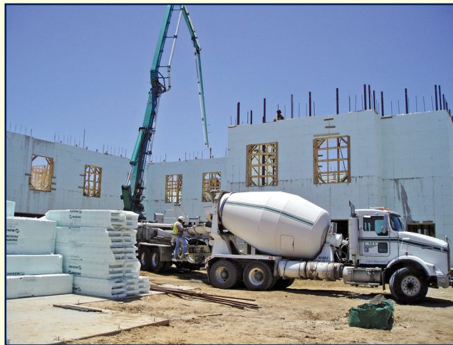
Figure 13 – Hilton Garden Inn, Lewisville, Texas, under construction. Images courtesy of Nudura.
