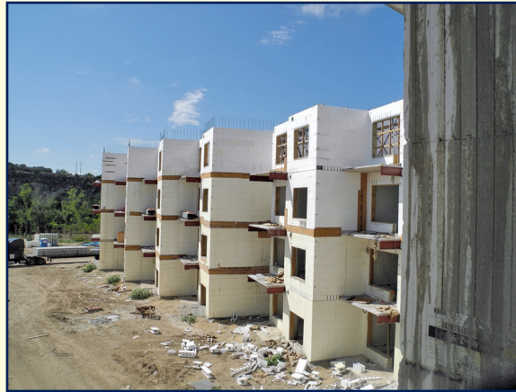
Figure 16 – The Ricchi condominiums under construction. Image courtesy of Fox Blocks.
