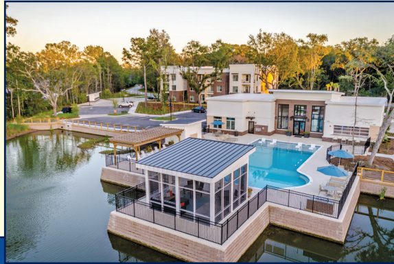
Figure 10 – 17 South Apartments. Image courtesy of EYC Companies.
