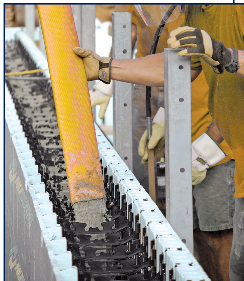
Figure 2 – Concrete being placed into ICFs. Image courtesy of Nudura.
