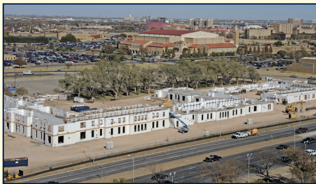
Figure 8 – West Village Student Housing under construction. Image courtesy of Fox Blocks.
