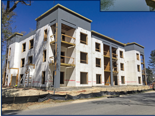
Figure 11 – 17 South Apartments under construction. Image courtesy of Amvic.
