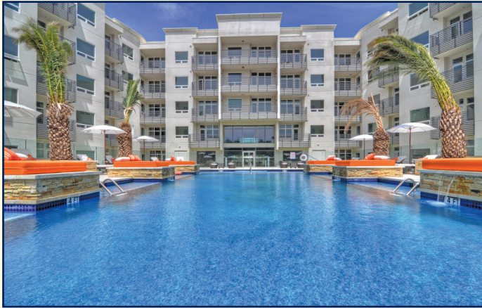
Figure 15 – The Ricchi condominiums. Image courtesy of Ricchi Group.
