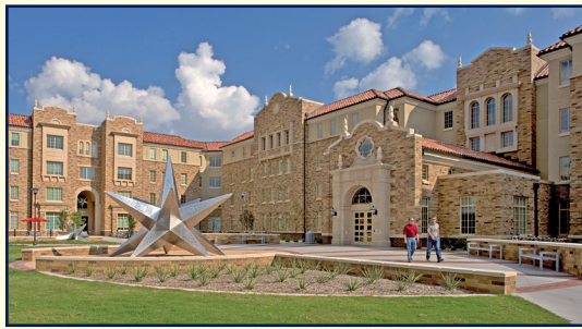
Figure 7 – West Village Student Housing at Texas Tech University. Image courtesy of Mackey Mitchell Architects.
