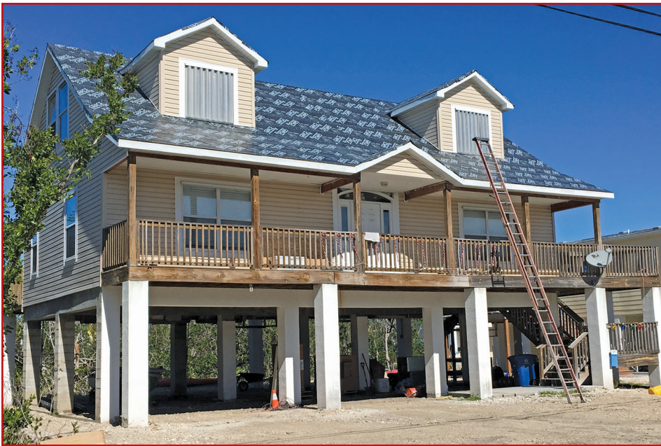
Figure 6 – Reroofing project using fully adhered underlayment. Courtesy of ARMA.
