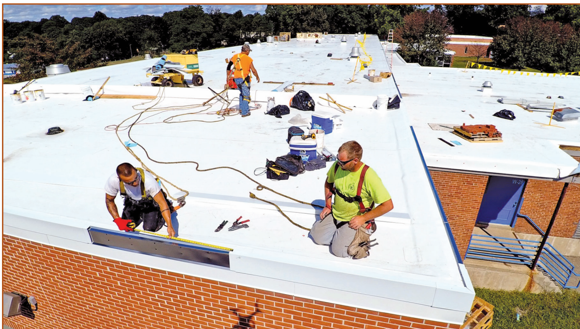
Figure 6 – ES-1 requirements are project-specific, which means that a product that meets the ES-1 wind design requirements for one building may not be appropriate for another building.
