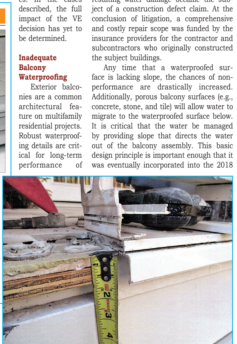
Figure 2 – As-built balcony details.
