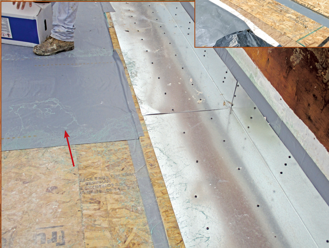
Figure 12 - Vapor/air barrier applied to field of roof.
