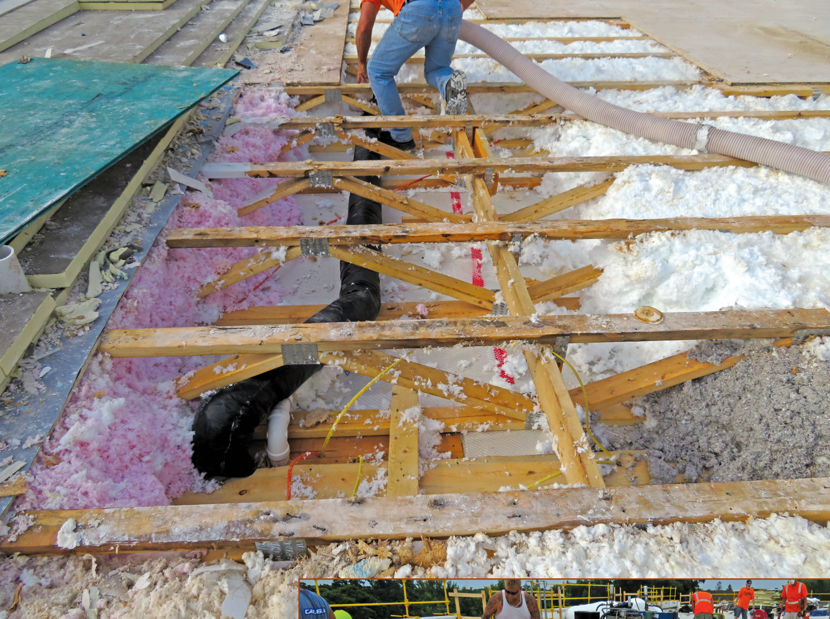
Figure 13 – Blown-in insulation.
