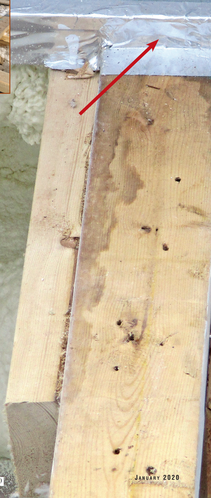
Figure 9 – Two-piece U-shaped vapor/air barrier transition metal.
