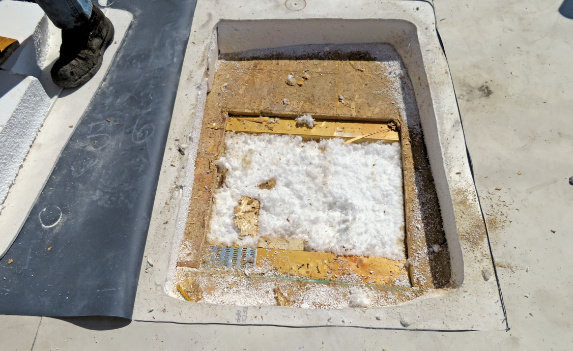
Figure 4 – Typical invasive inspection opening above trusses.
