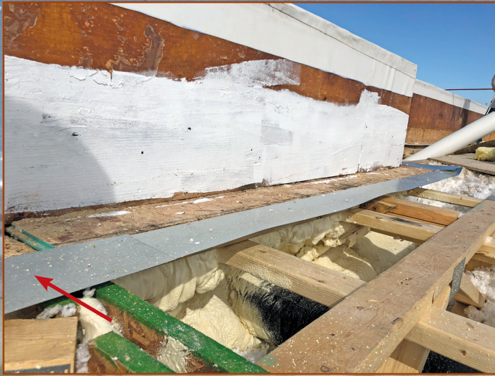
Figure 8 – Z-shaped vapor/air barrier transition metal.
