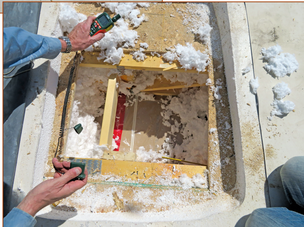
Figure 5 – Typical invasive inspection opening below roof deck sheathing.
