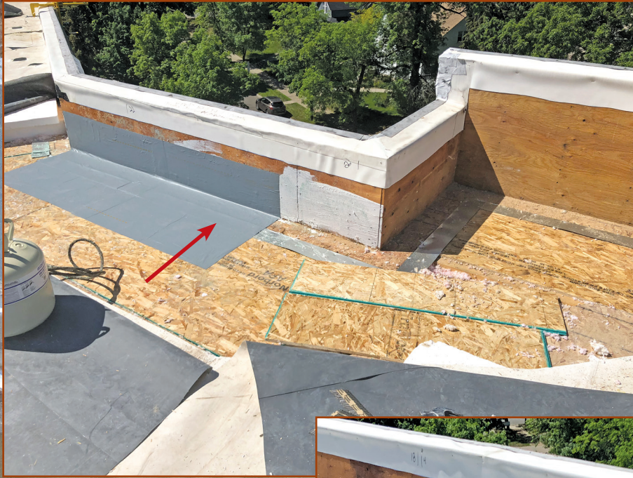
Figure 10 - Roof vapor/air barrier at roof perimeter.
