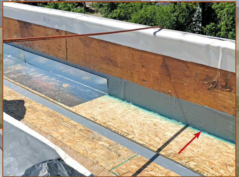
Figure 11 - Plywood and sheet metal angle parapet reinforcement.
