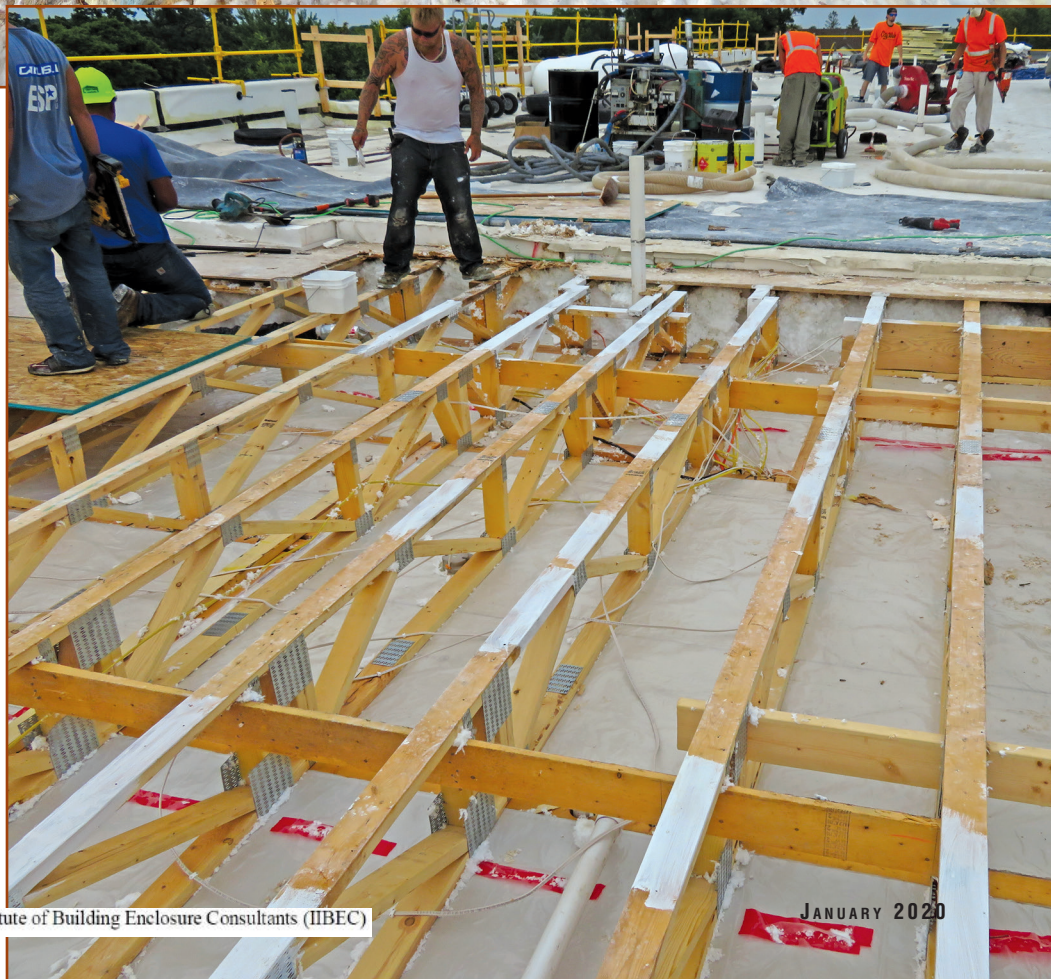
Figure 14 – Mold remediation paint.
