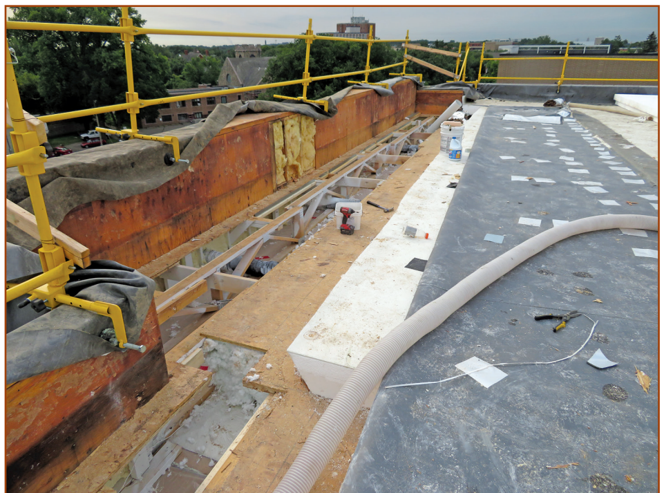
Figure 7 – Typical work at roof perimeter.
