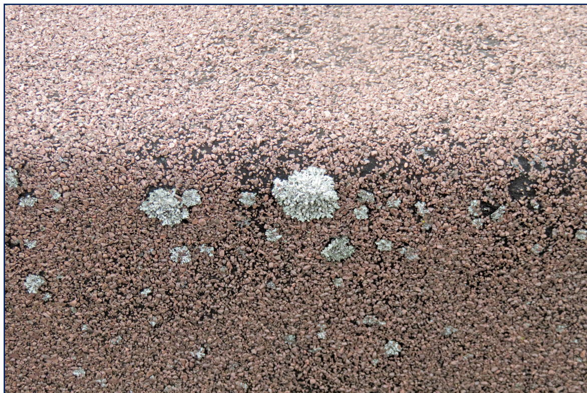
Figure 5 – A close-up of one patch of lichen. It does not look anything like moss.
