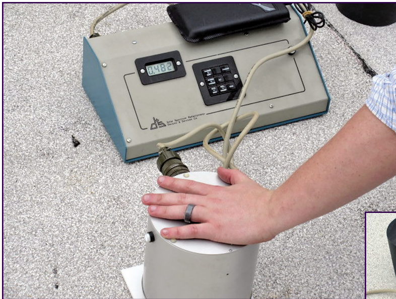
Figure 13 – Reflectivity reading of 48 on cap sheet with stained granules.
