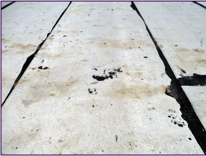
Figure 3 – “Cool” roof cap sheet applied in hot asphalt.
