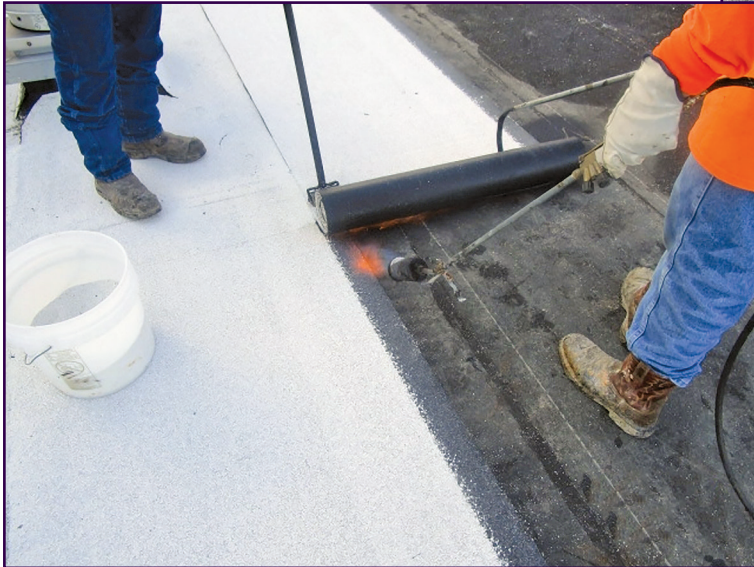
Figure 7 – Torch application of white-colored granule-surfaced cap sheet.
