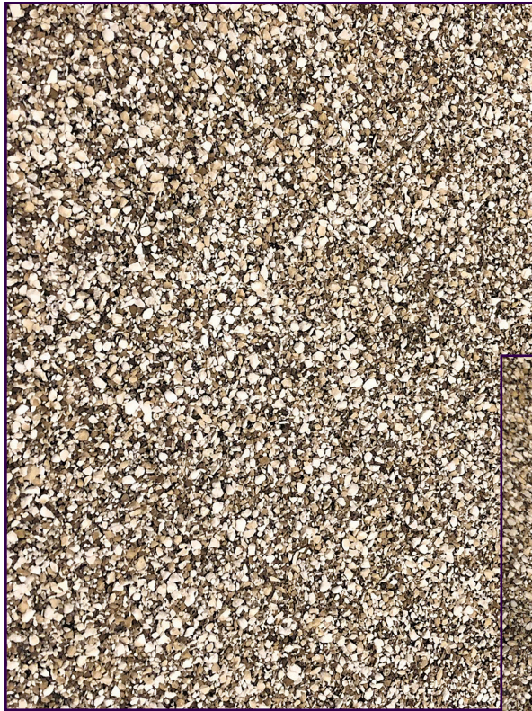
Figure 10 – Close-up of stained white-colored granules of cap sheet.
