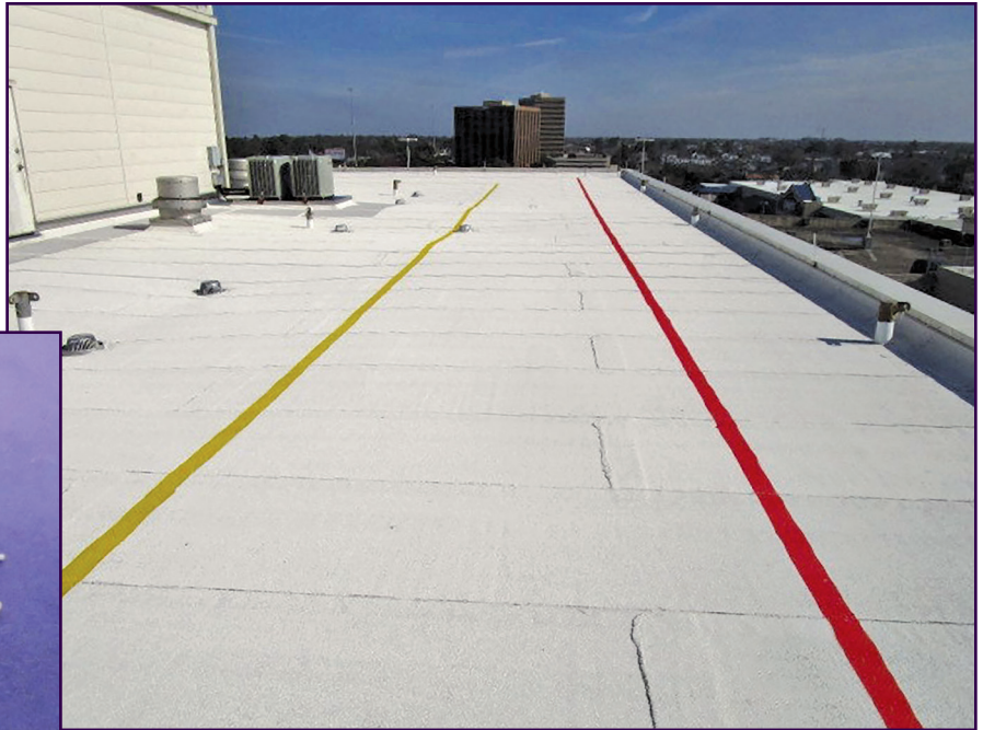
Figure 17 – Overview of installed white-colored granule-surfaced cap sheet.
