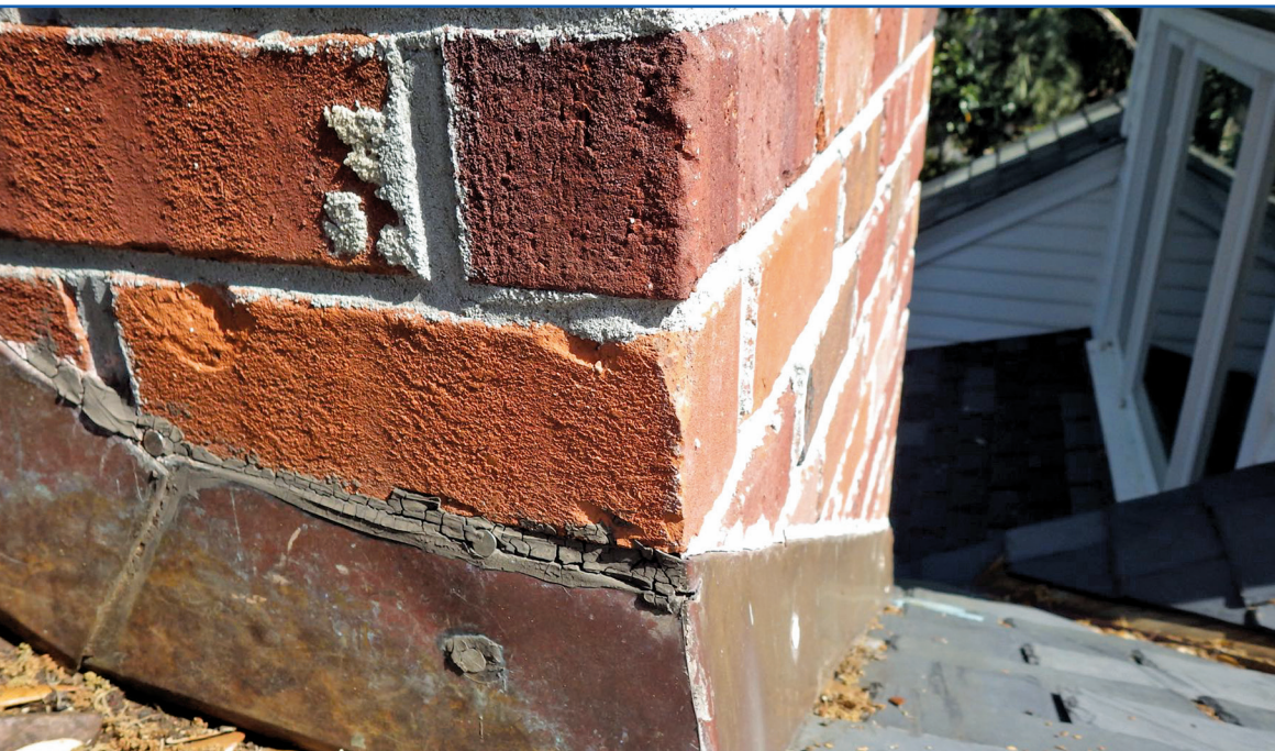
Figure 5 – Typical surface-mounted flashing.
