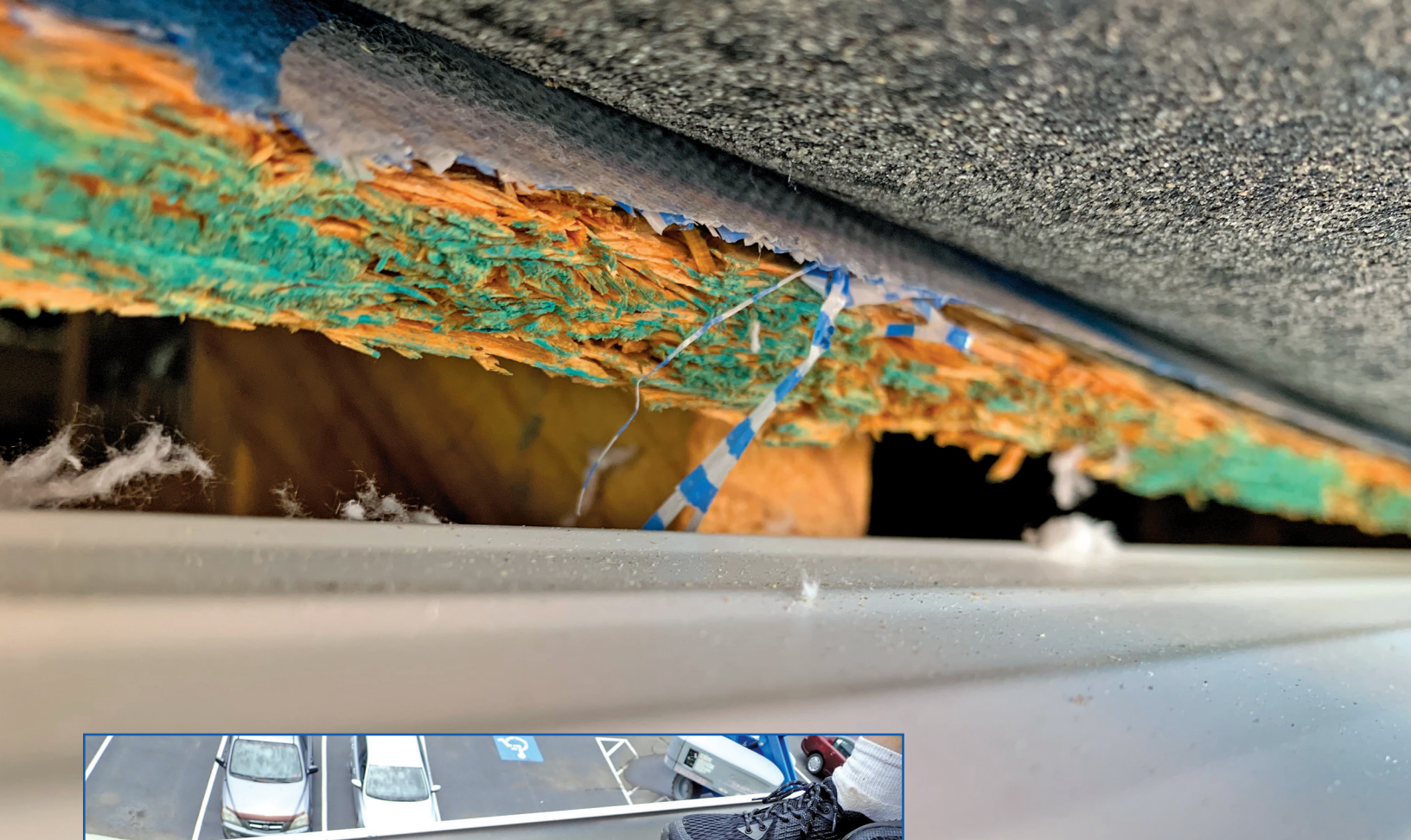
Figure 13 – Improper eave flashing.
