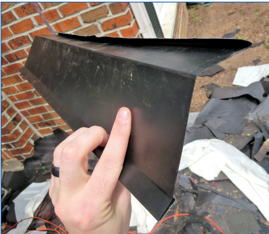
Figure 12 – Profile view of best-practices counterflashing.
