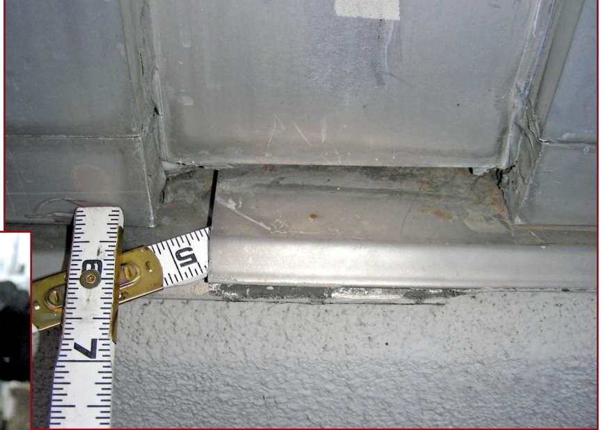
Figure 8 – No sealant installed in flashing lap.
