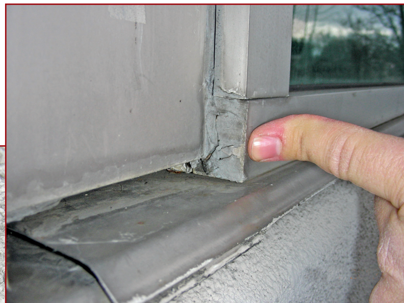
Figure 6 – Sealant pumped into open end of sill component extrusion.
