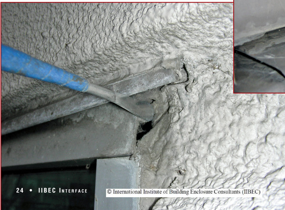
Figure 4 – Removal of finishes at metal stud track directly below windowsill revealed water staining and corrosion of fasteners.
