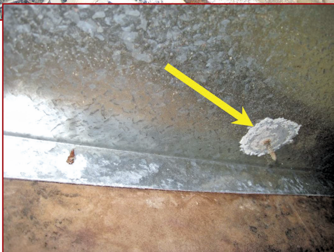
Figure 4 – Removal of finishes at metal stud track directly below windowsill revealed water staining and corrosion of fasteners.
